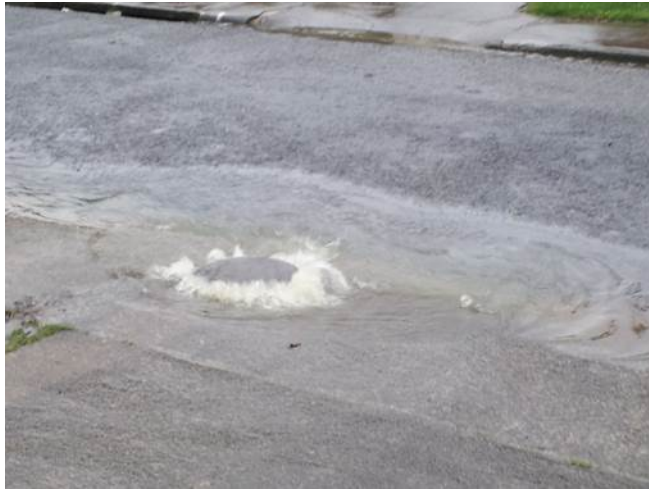
Figure 3: Another example of surcharging wastewater manhole
