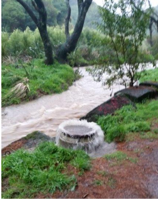
Figure 2: Surcharging wastewater manhole in Porirua during heavy rainfall
