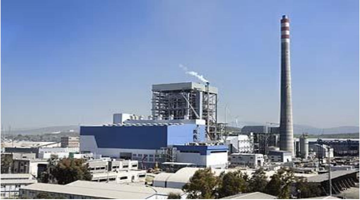
Resim C.1 – İzmir Enerji Termik Santrali (Google, 2018)
