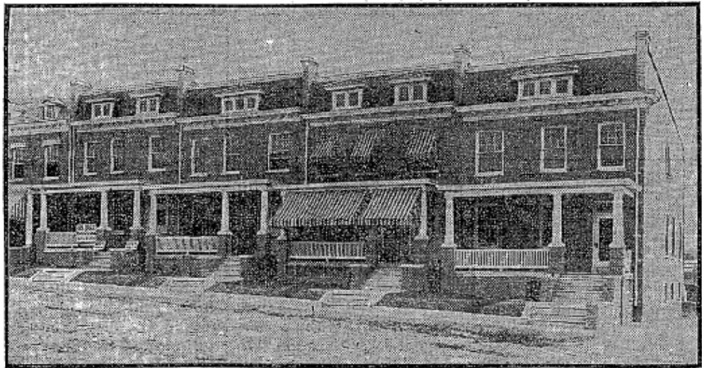
A row of four houses in Fifteenth street, near Webster street northwest, has recently been completed by W. C. Allard. They are at No. 4407, 4409, 4411 and 4413 Fifteenth street. The buildings are two stories high, and are built of light brick. There is a block style cement porch extending across the entire front of each building, and a double back porch inclosed in glass. The houses are 23 feet wide. An expenditure of about $25,000 was made in erecting these dwellings.
