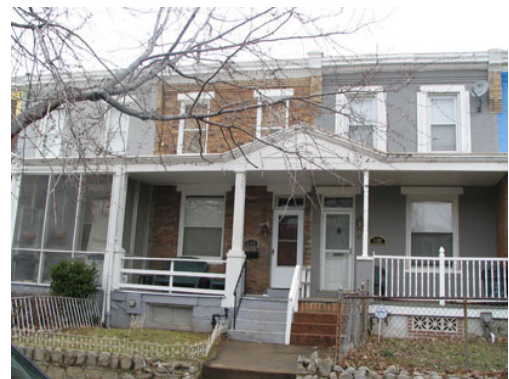
1620 G Street, SE with front porch rowhouse design EHT Tracerics, Inc., 2010
