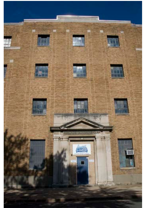
Arcade-Sunshine Cleaning and Laundry Plant; 735 Lamont St., NW EHT Tracerics, Inc., 2010
