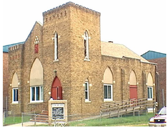
St. Paul AUMP Church, 401 Eye St., S.E., 1924 District of Columbia Office of Planning, 2004
