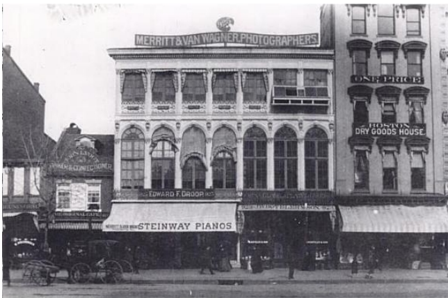
Iron Hall, 925 Pennsylvania Avenue, NW, 1851. Cast-Iron Architecture in America, 109.
