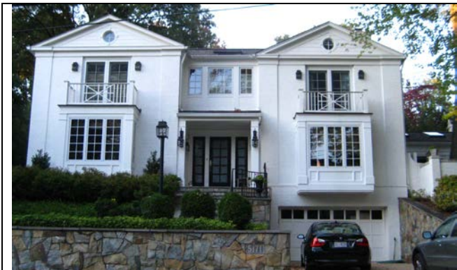
5171 Manning Place, N.W. Kirkhuff & Bagley 1941 EHT Traceries, 2010
