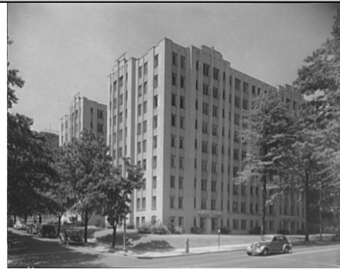
Apartment Building, 2000 Connecticut Avenue, NW. Library of Congress, LC-814-T-2391-046
