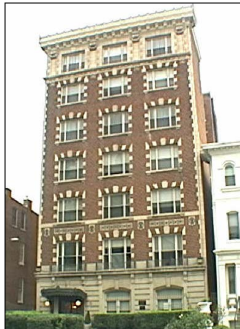
Apartment Building, 1509 16 th Street, NW. Averill, Hall & Adams, 1909.
