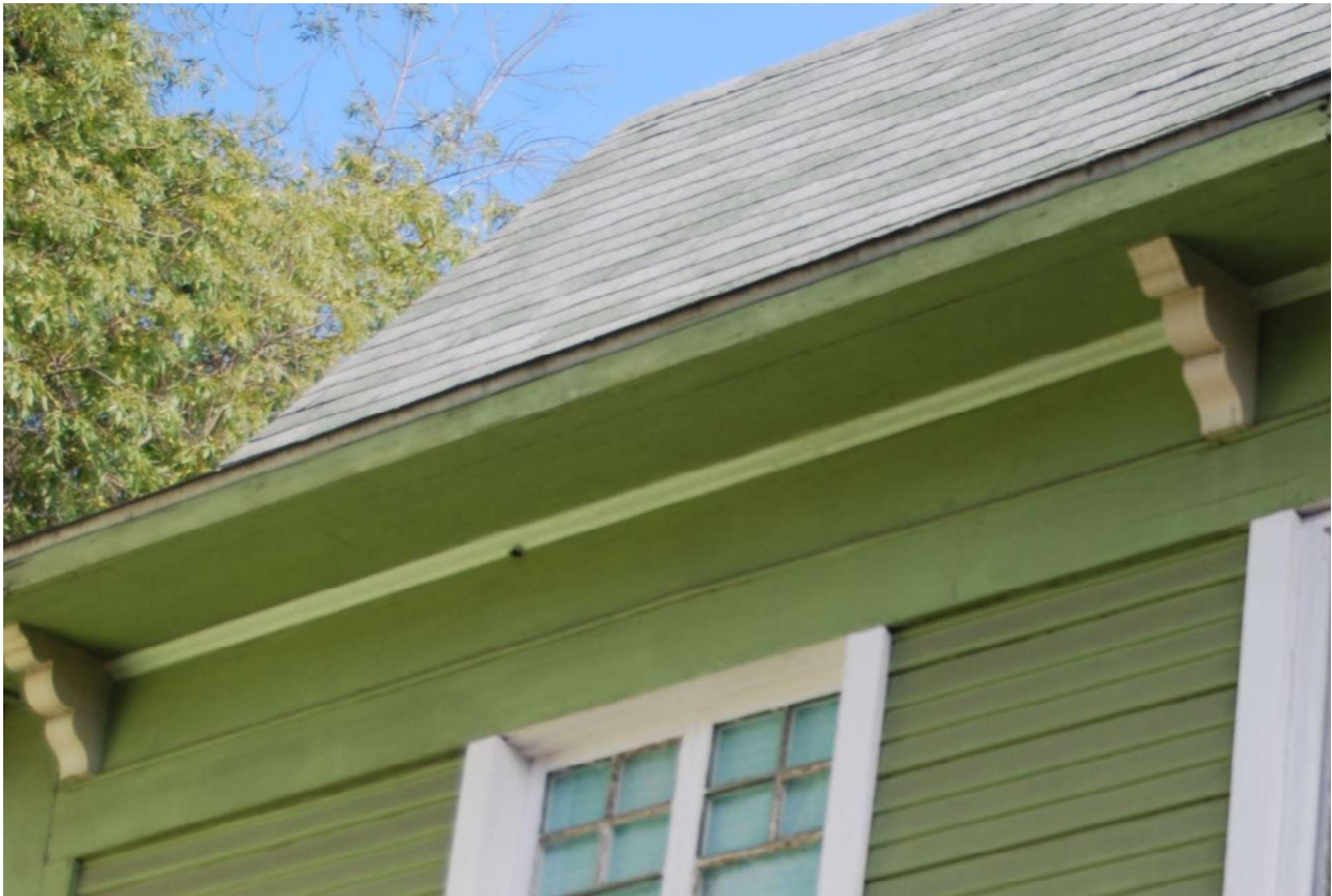
Queen of Elysian Heights, enclosed eaves & brackets, 1553 W. Ewing Avenue, November 22, 2021 (Photo by Charles J. Fisher)
