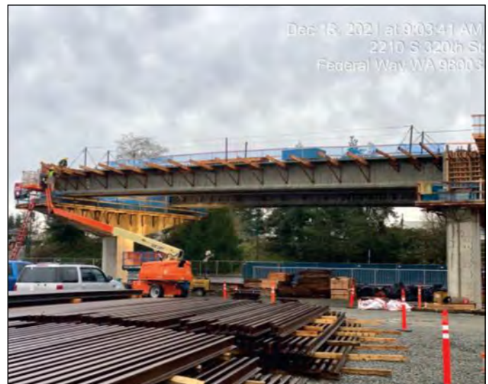
WA3.8 Overhang Decks Span G18
