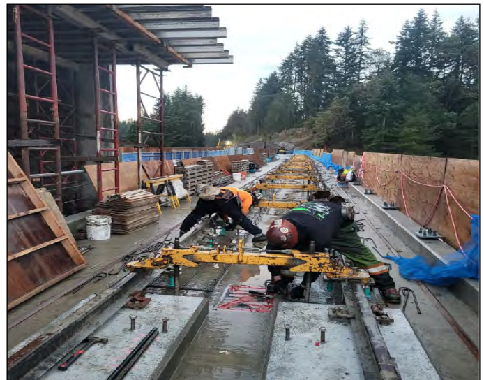
Trackwork and plinth installation at MLT station.
