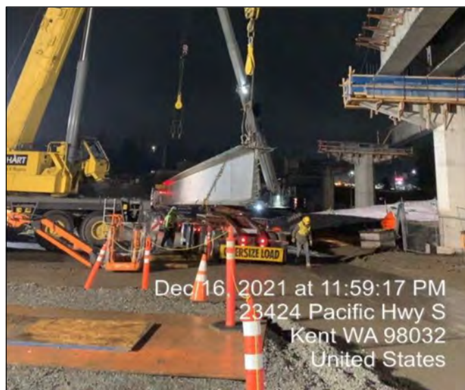
WA1.3 Girder Plcmt KDM Rd. Close OL
