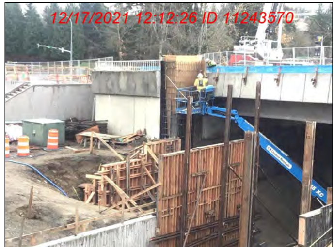
The carpenter working on the wall form at the pedestrian crossing.
