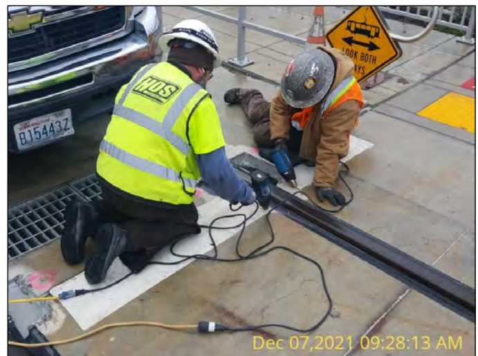
Boot repair holes dried prior to grout placement facing south.
