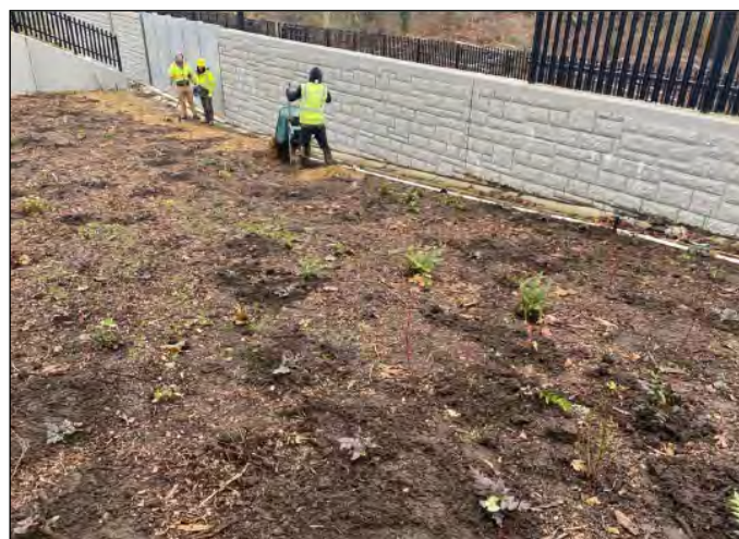
Final mulch placement along embankment adjacent to the Winter's House
