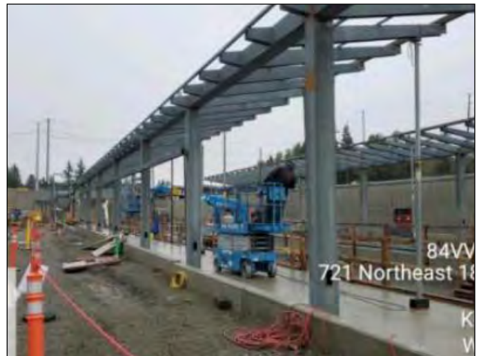
185th station canopy steel
