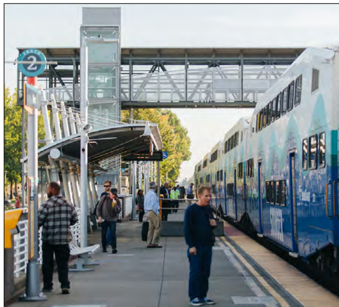
Improving access to Sounder Kent Station
