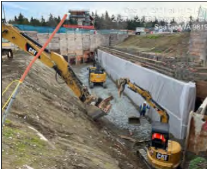
WA 1.1 Pier 3 Backfill Progress
