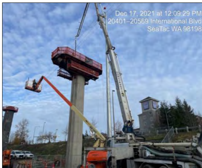
WA1.1 Cap A08 Concrete Placement
