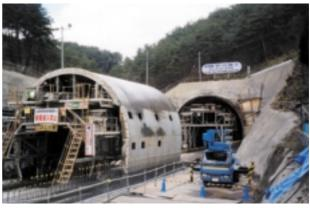
Photo 2. Movable form placed at the Tokyo portal of the Midou section
