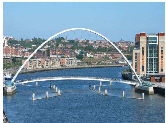
Figure 4: Cables merging into the background
