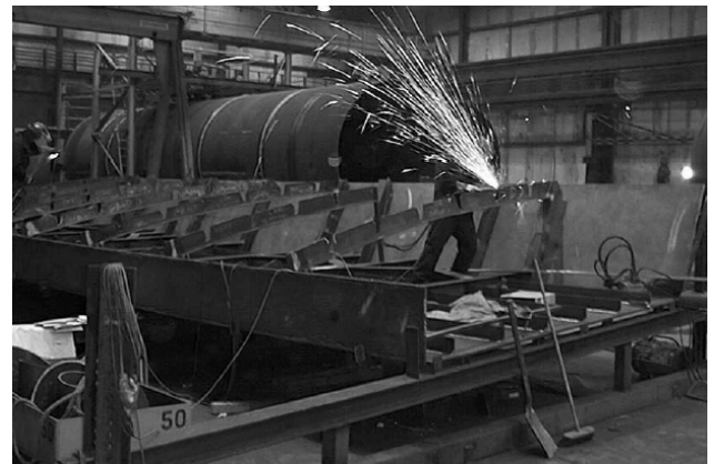
Figure 6: Construction of the deck
