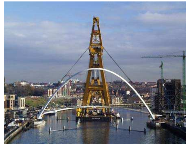
Figure 7: Lifting the bridge onto its supports
