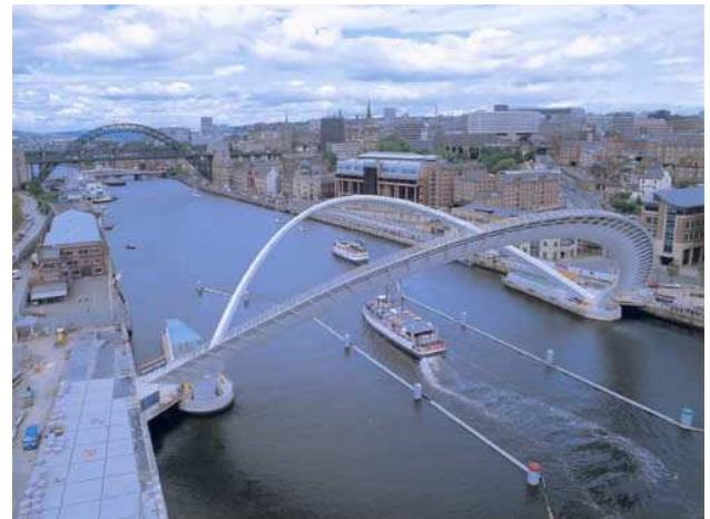
Figure 2: The Bridge in its open position
