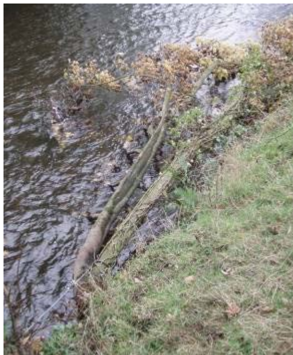
Photo 10 Tree anchored to its stump by cabled wire
