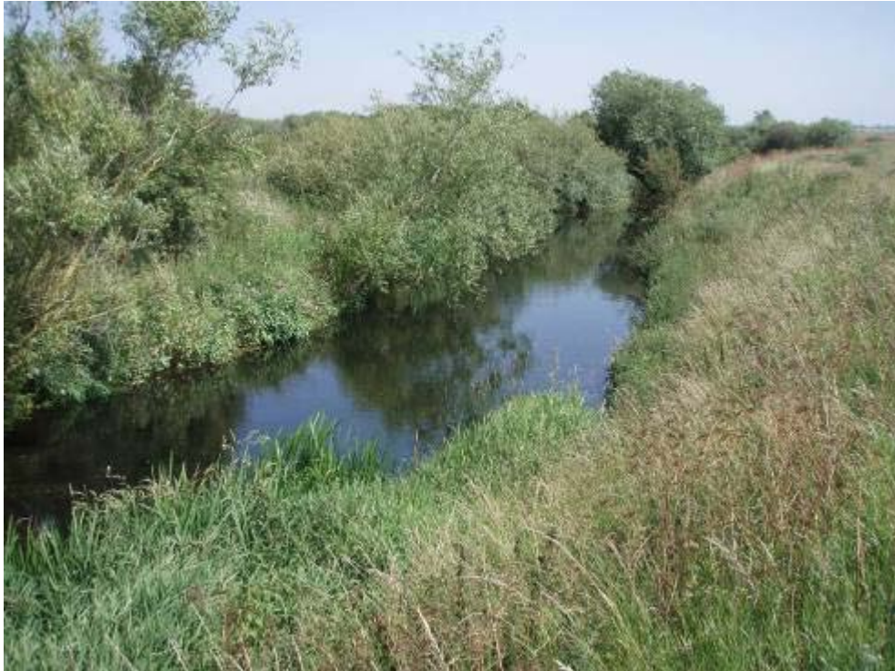
Photo 1 Reasonably good cover is provided by the overhanging willows on this section
