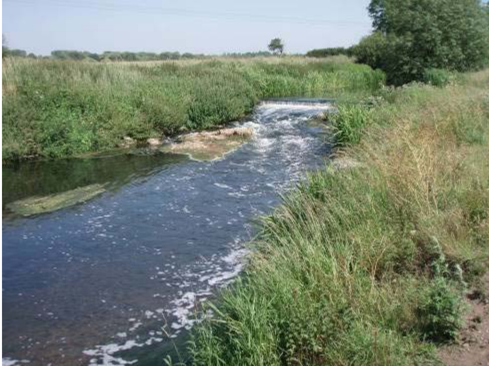
Photo 8 The weir the function of which is reportedly to control water levels in Retford upstream (despite the propensity for flooding there....?)
