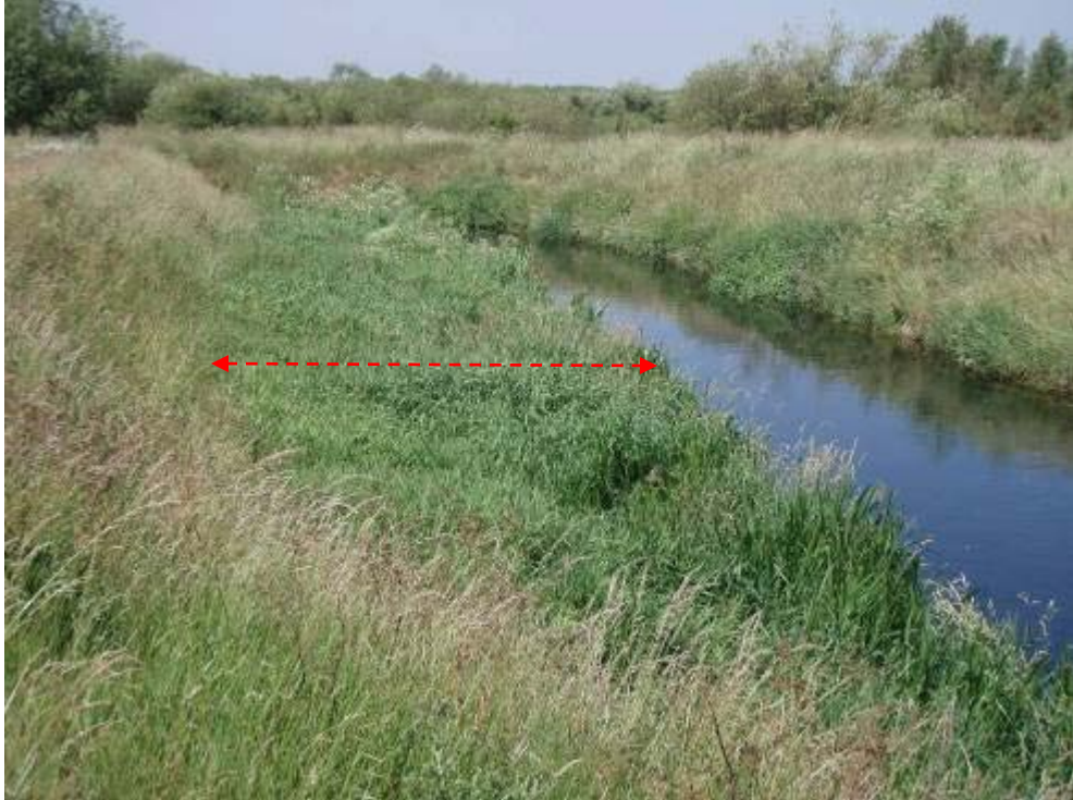
Photo 11 Existing berm on the Idle upstream of Chainbridge Lane
