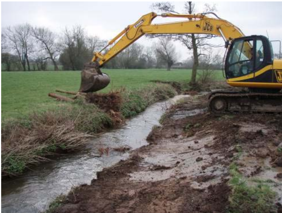
Photo 12 Bank re-profiling on the inside of a bend
