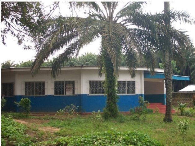
RTC Main Building
