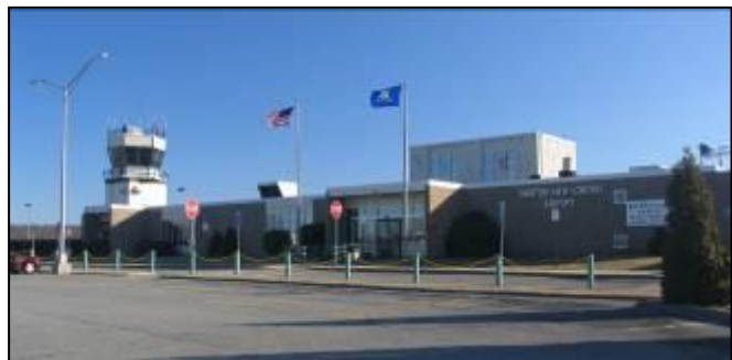
Figure 2.10 – Terminal Building (Landside)
