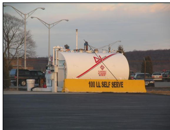
Figure 4.3 – Self-Service Fuel System
