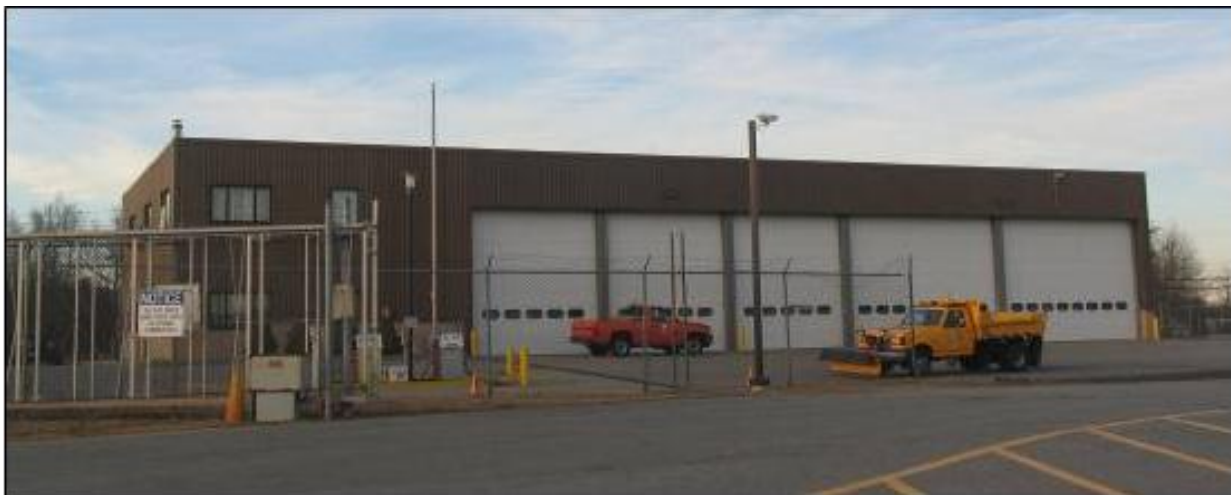
Figure 2.13 – SRE Storage and Airport Maintenance Building
