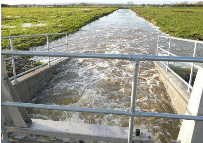
Operation of new IDB inlet – winter 2009
