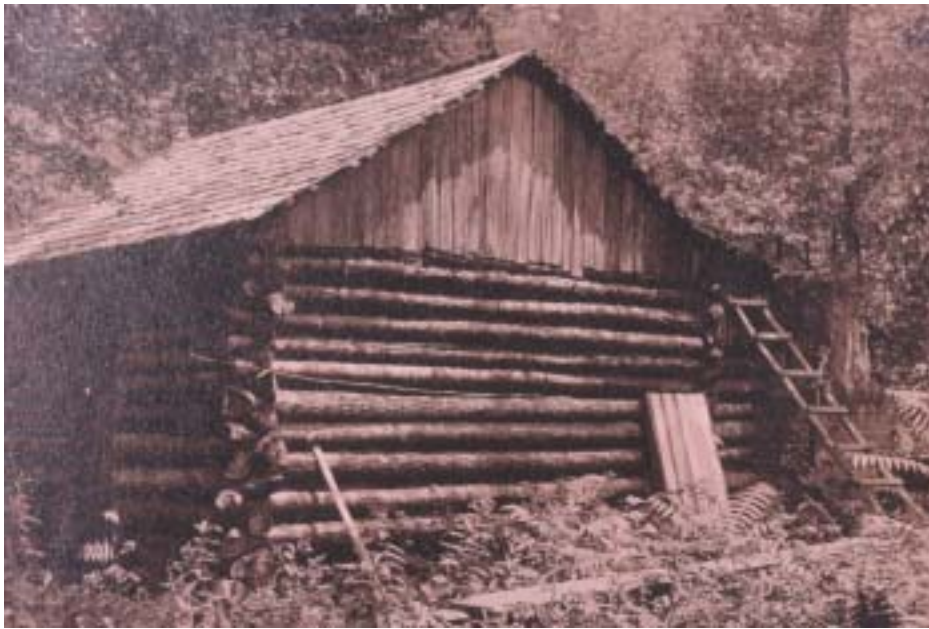
Figure 15: Unknown House. “Chimney Under Construction.” Courtesy Ouachita National Forest.
