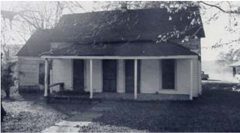
Figure 21: Residence #1, Caddo Gap, Montgomery County. AHPP Photo.
