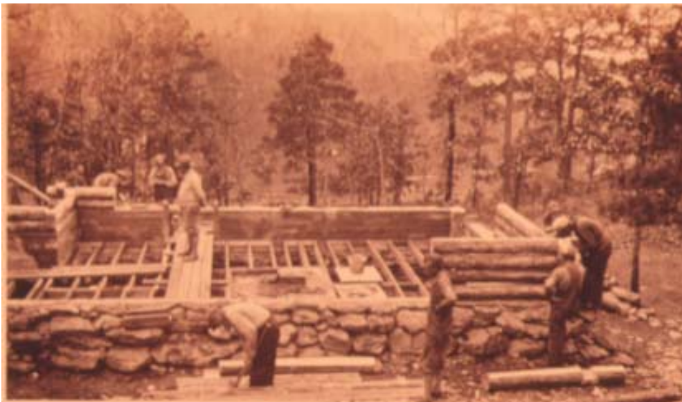
Civilian Conservation Corps workers build a cabin at Petit Jean State Park. Courtesy of Arkansas Department of Parks and Tourism.
