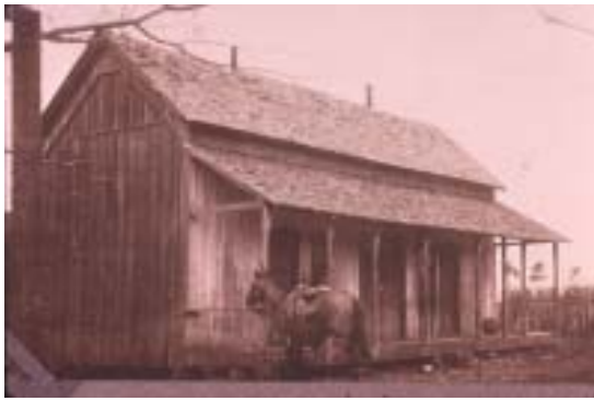
Figure 17: Unknown Structure/Ranger Station? Courtesy Ozark-St. Francis National Forest.
