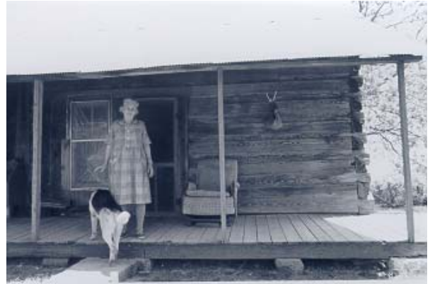
Figure 20A: John Vickery Homestead (ca. 1904), Fiftysix vic., Stone County. AHPP Photo.
