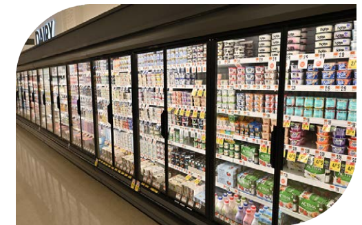
Remodeled Stop & Shop store with new refrigerant system.
