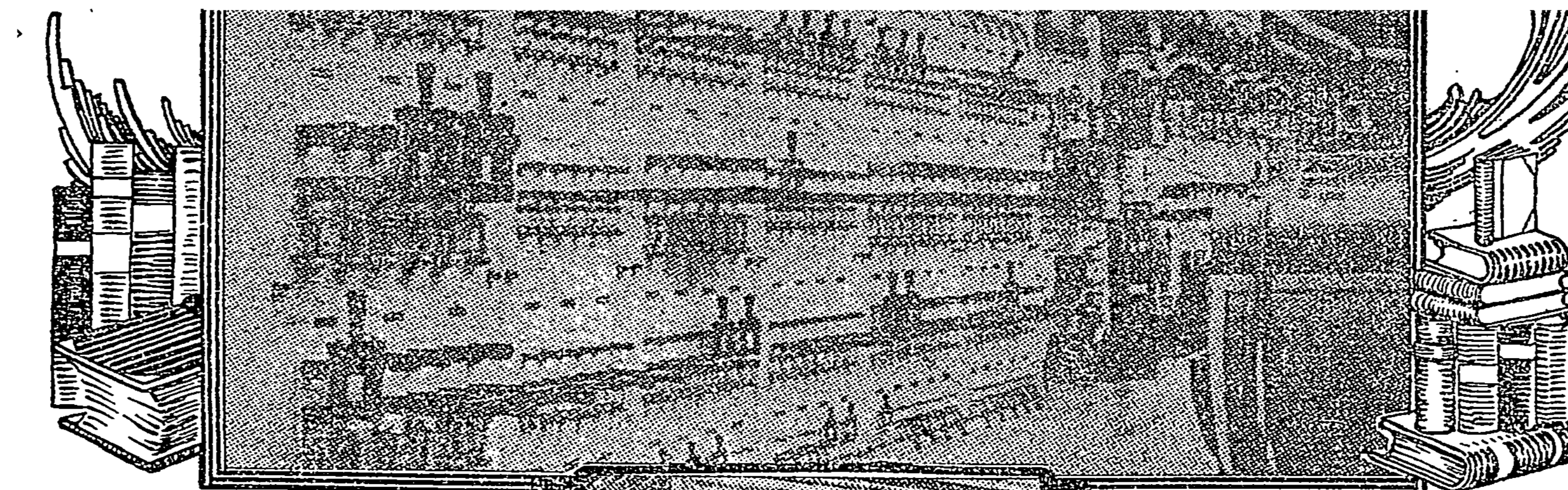
Marble switchboard which controls the electrical appliances of the building.
