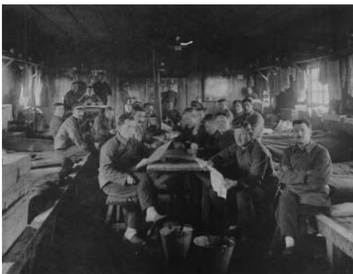
Inside of Captives' barrack
