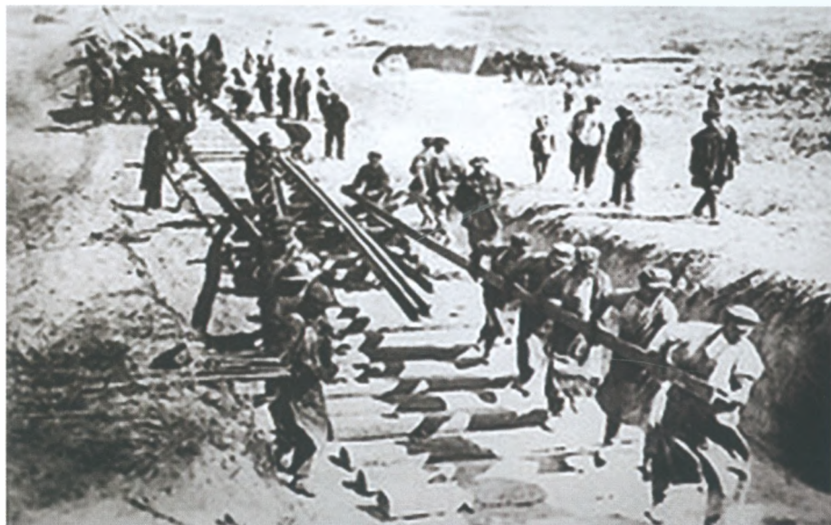
Workers building the Sakhalin Railway in the 1930s. Railway construction was arduous and often dangerous work.
