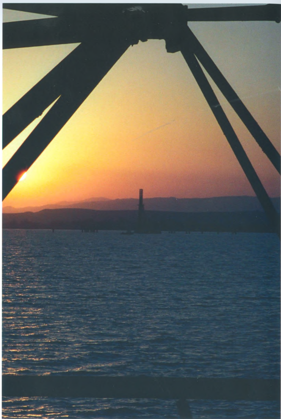
The jetty of the BTC final terminal, a pipeline that would transfer oil from Azerbaijan to Turkey and on to European markets.
