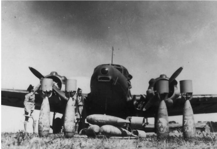
Anson crews at Mallala pose cleverly with 100-pound anti-submarine bombs in March 1942 to make them look man-sized. At this time other RAAF aircraft usually used 250-pound bombs but such weapons were too large for the Anson which had only a very modest bomb carrying capability. Messages and drawings for their Japanese recipients can be seen on the bombs, with the one on the far right reading "FROM 70 SQN". (George Robertson via Mallala Museum)
