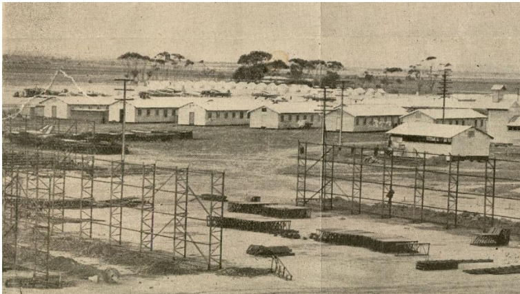
A newspaper photo of the Mallala base in 1941. Many huts have been erected, but some are still incomplete. In the foreground the assembly of a Bellman hangar has commenced. Several Ansons are visible at the top of the photo, dating the picture at September 1941 or later. (Mallala Museum)
