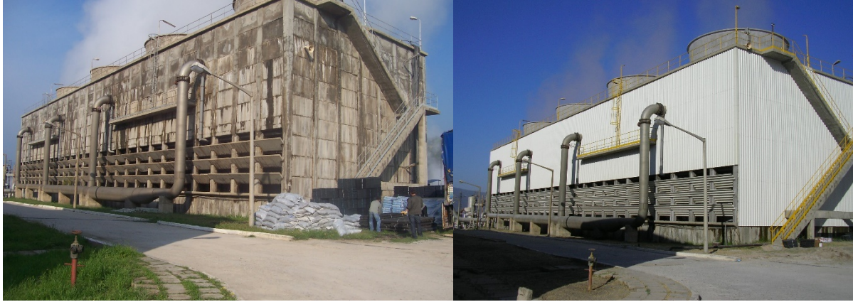
Figure 3: KZD-1 cooling tower before and after retrofit.
