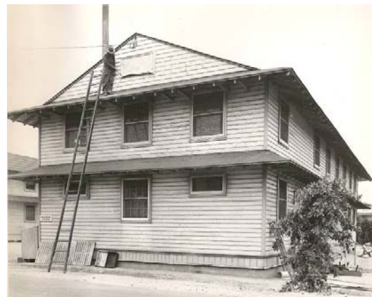
Figure 4: Wedging the widows shut (top) and sealing the louvers (bottom).
