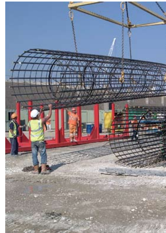
Express Reinforcements Ltd.
