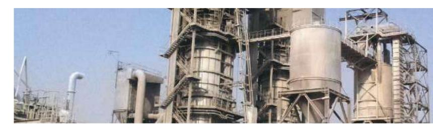
With the support of a diligent team, Lime Calcination Plant was commissioned in Qatar Steel on December 2011 for producing calcined lime and dololime for captive consumption. Both high calcium and dolomitic lime enjoys its most extensive use as a flux in refining of the steel in EAF. Lime is particularly effective in removing phosphorus, sulphur, and silica, and, to a lesser extent, manganese.
