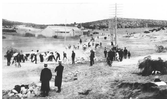
Figure 20 Repairing the Perth to Fremantle Road, 1914.
