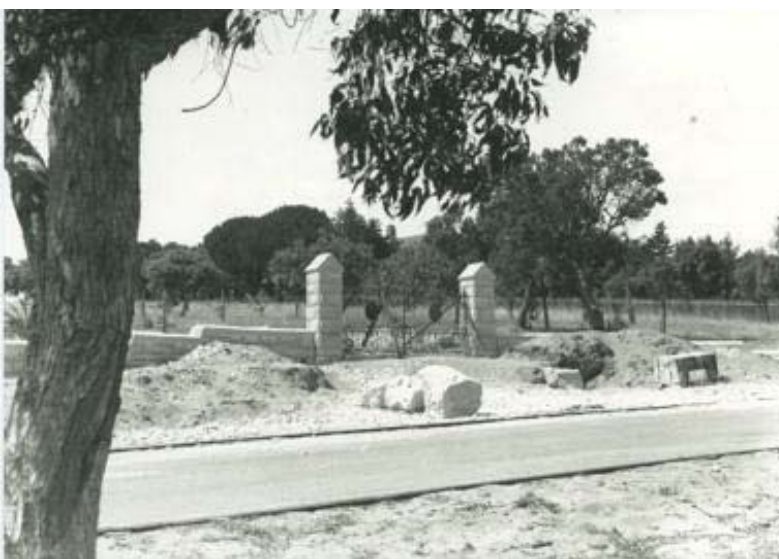
Memorial Gates Palmerston Street, 1935, courtesy the Grove Library CPM01127
