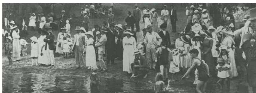
Figure 19 Celebrating the construction of the foreshore road, 1914.
