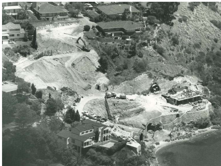
Figure 31 Ground works for new residences at the Chine, 1989.
