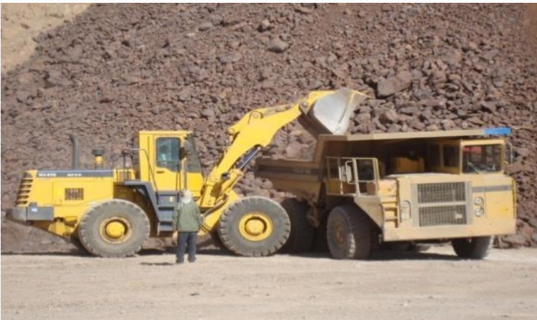
EXCAVATING AND, HAULING by 100 t trucks
