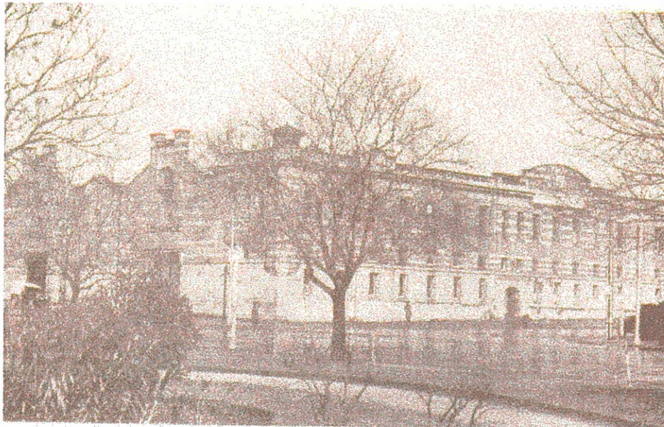
The Grenfell Street Power Station in 1946. This picture appeared in “Fifty Years of Progress”, the book produced by the Adelaide Electric Supply Company to commemorate its 50 year history.
