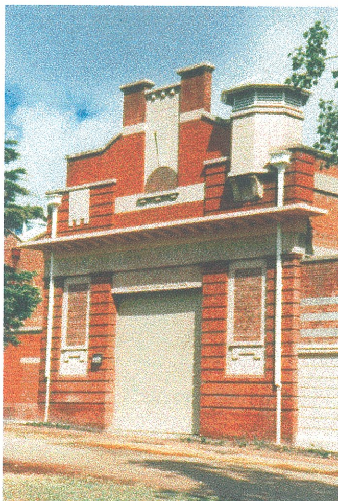
The Adelaide Electric Supply Company Converter Station
