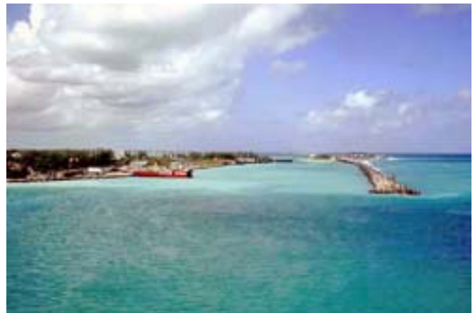
Arawak Cay—West Breakwater
