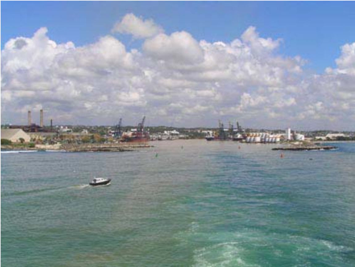
Puerto de Haina Entrance
