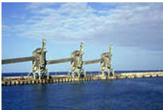
Bridgetown—Conspicuous Sugar-loading Towers
