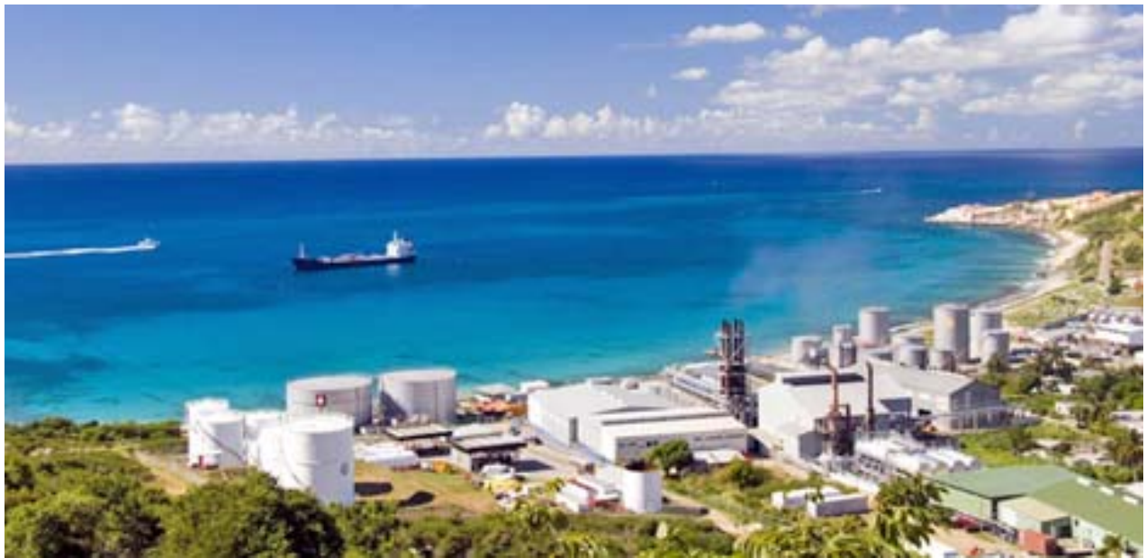
Cole Bay Oil Terminal
