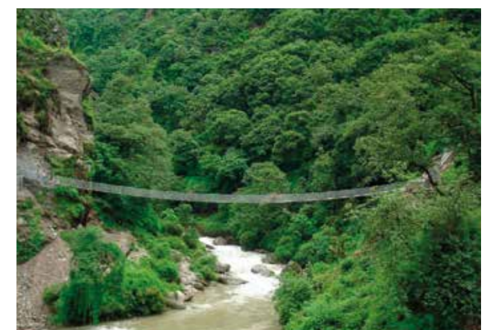
A suspended bridge (64.5m) over Urimpar Khola between Sertung and Lapa VDCs of Dhading
