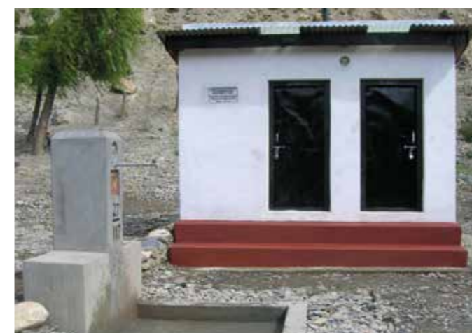
RSWP Water project with a two room latrine
