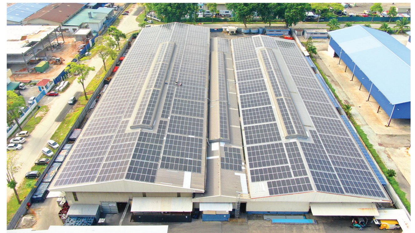
In FY2020, the solar power system at our Factory 18 supplied 1.26GWh of green energy to glove manufacturing, representing savings of 874.44 tonnes of CO 2 and RM500,000 per annum.
