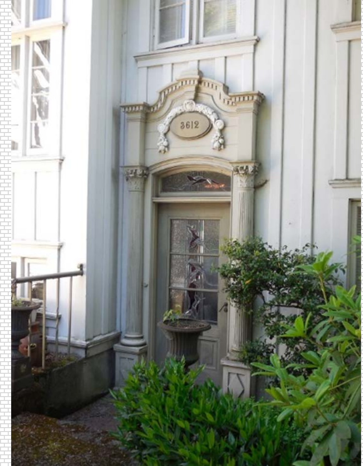
Egil Mack Residence, 1917 3612 E. Union St., Existing
