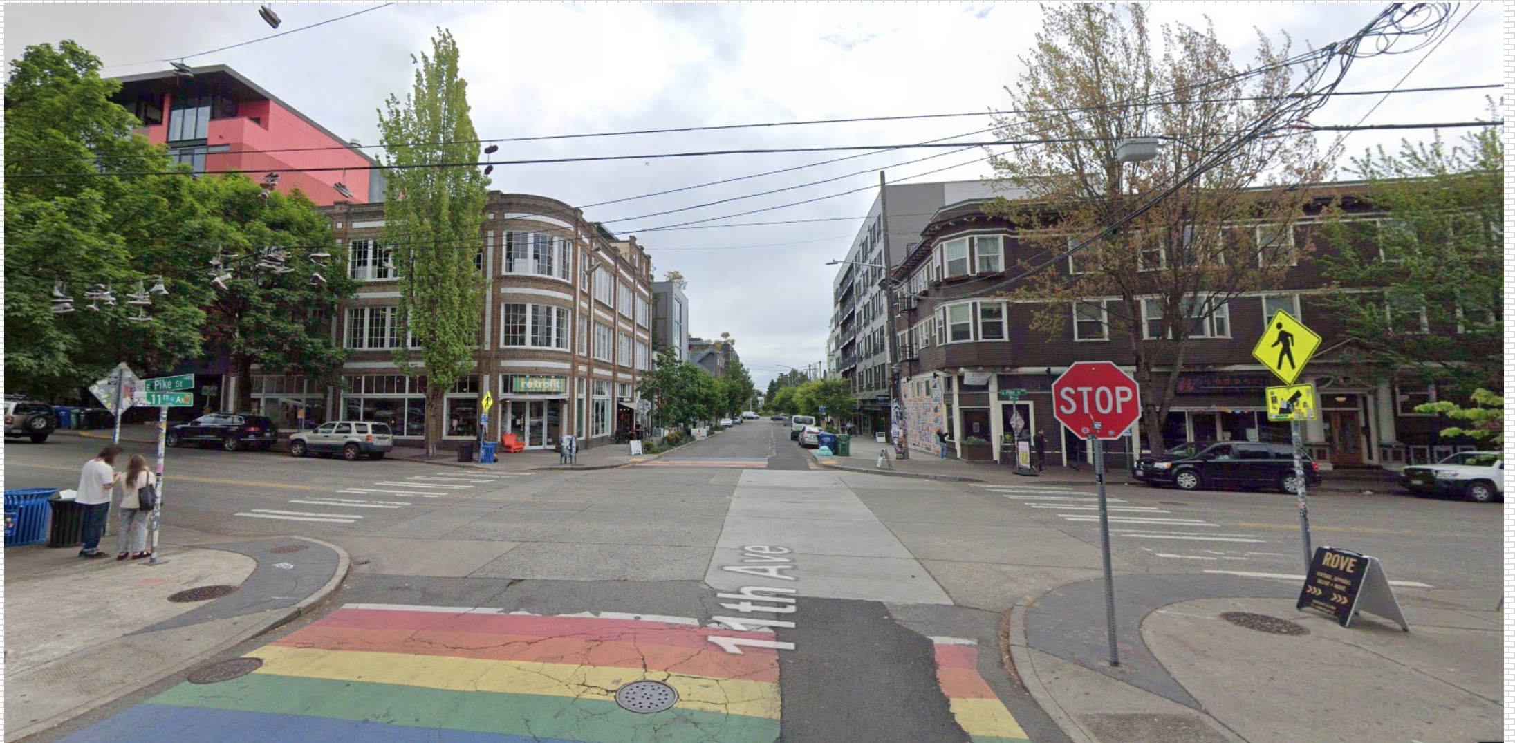
Figure 2) Context photograph of subject building looking south down 11th Avenue. (Google)
