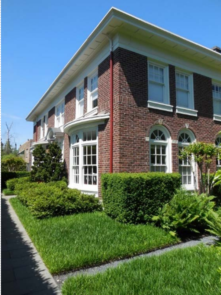
Perry Truax Residence, 1915 951 Federal Avenue, Existing
