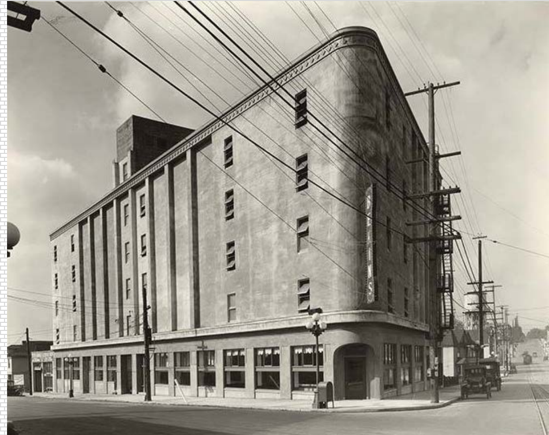
Bekins Moving & Storage Warehouse, 1918 1125 12 th Avenue East at East Madison, Seattle , altered
