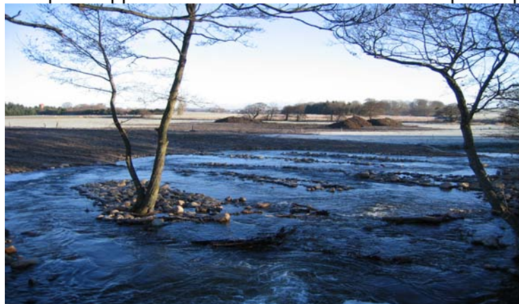
The lower segment of the new stone riffle
