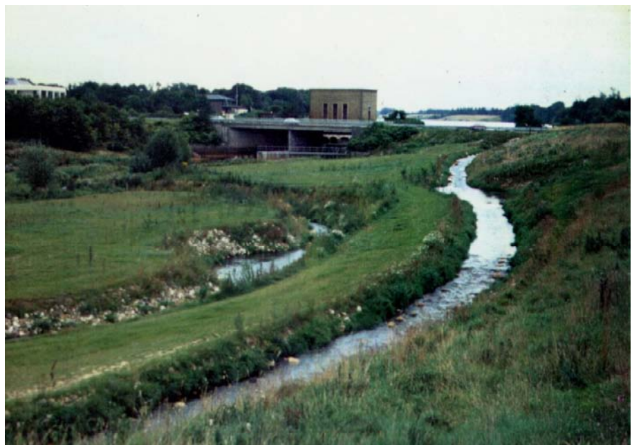
Spawning ground in the uppermost reach of the bypass riffle. In the background can be viewed the hydroelectric power station and its lake.
