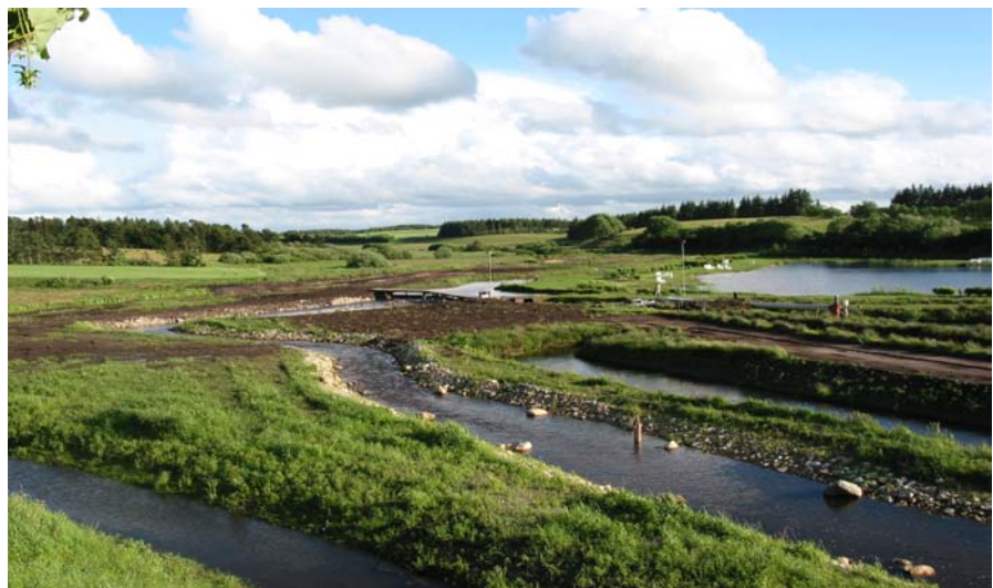
The new fish pass at Munkbro Fish Farm in the river Vegen
