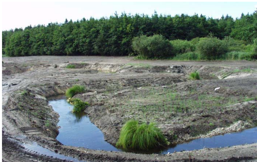
Digging the new meanders
