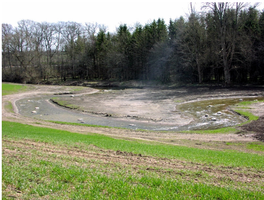
A new meander with a 3.5‰ slope
