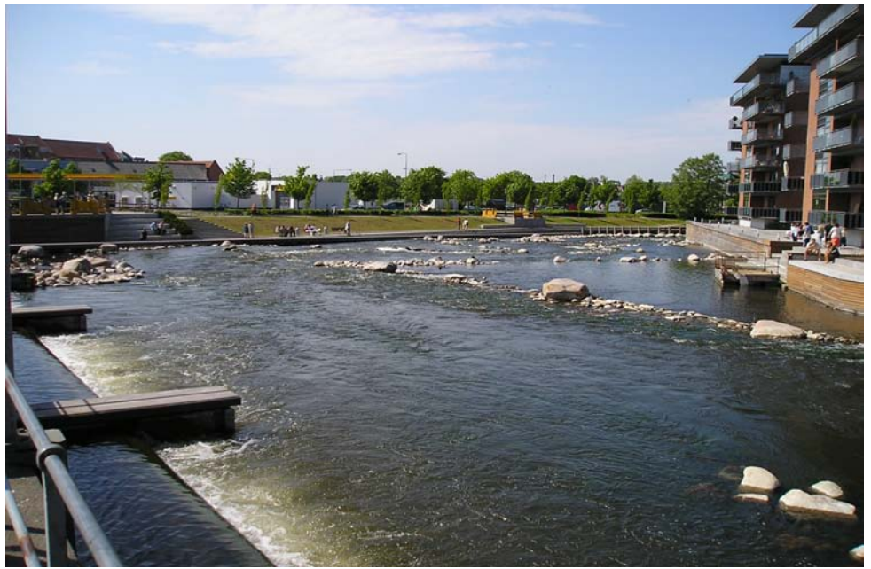
The new weir and the fish pass viewed from downstream
