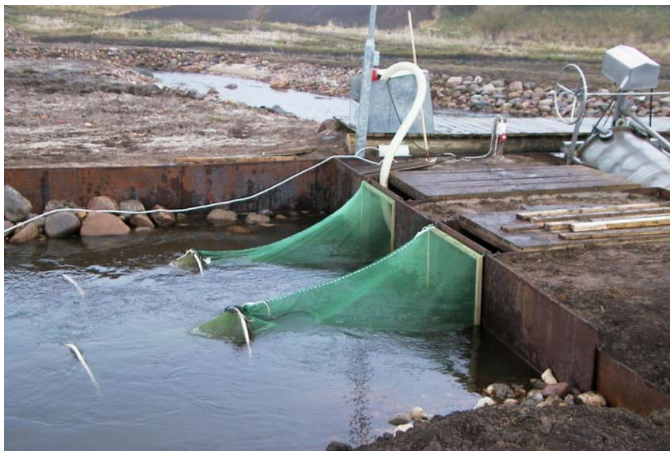
Fish traps in the intake to the fish farm. The biodrum screen can be seen on the right, and the riffle in the background
