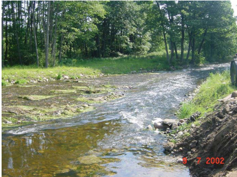
The current channel and overflow basin.
