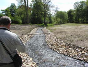
Newly established stone riffle
