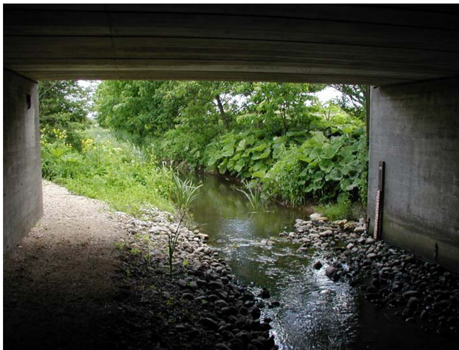
Motorway bridge at Jersie Mire
