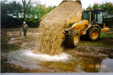
Spawning gravel being laid out
