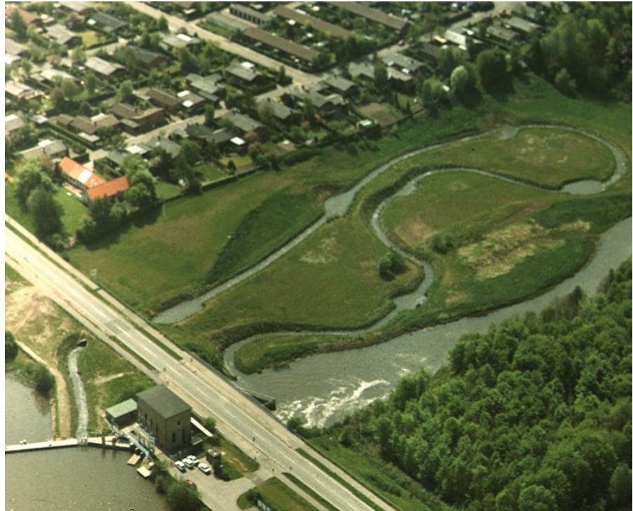
Aerial photograph of the hydroelectric power station during a situation with high flow through the sluice and turbine
