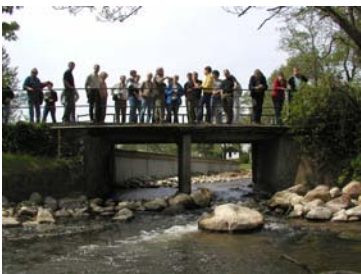
After removal of the weir
