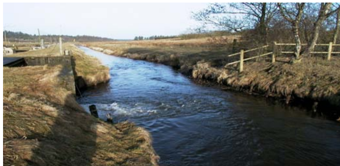
Prior to alteration of the fish farm's outlet
