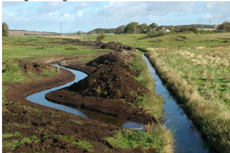
The meanders during excavation
