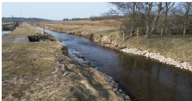
After alteration of the fish farm's outlet
