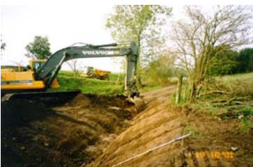
Digging from the side
