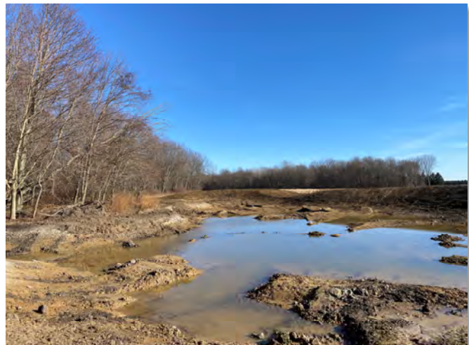
A 0.5 acre wetland was created in a wet area of an agricultural field adjacent to a woodlot containing a provincially significant wetland feature.
