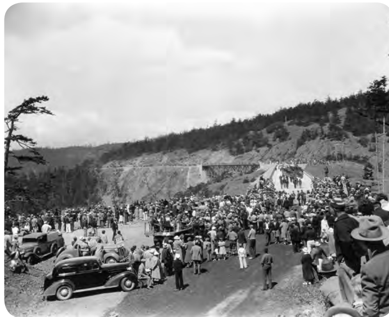
right Deception Pass Bridge dedication, 1935, looking north. SR 20. Source: Washington State Archives.
