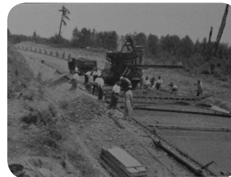
this page 1938-1940 view of Muck Creek Hill (SR 7), paving revised grade with concrete. Source: Washington State Archives.
