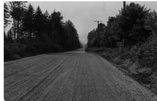
1997, Skykomish River Bridge vicinity (between Gold Bar and Reiter) work approved
