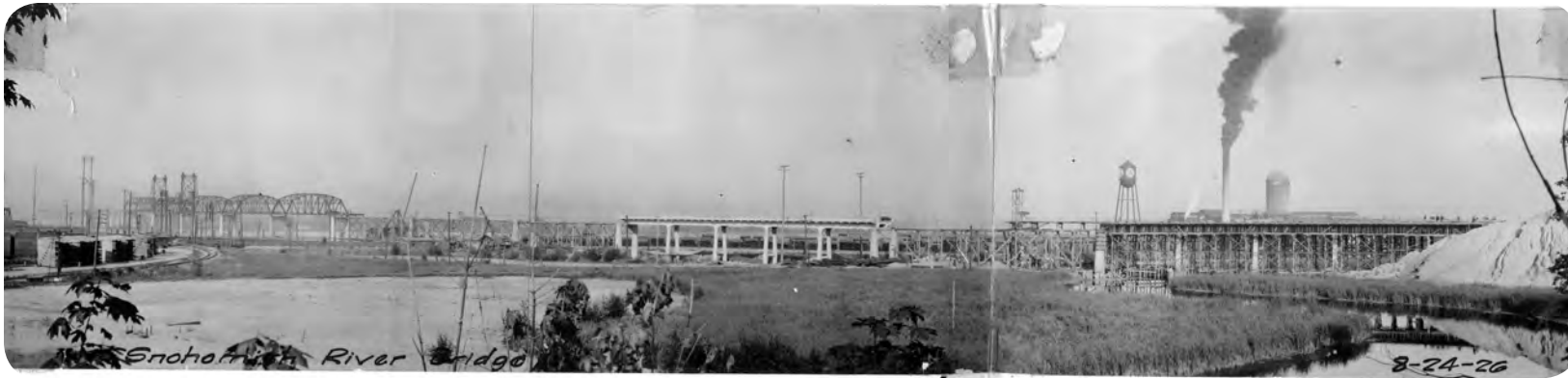
top 1926 view of Snohomish River bridge (SR 2). Source: Washington State Archives.
