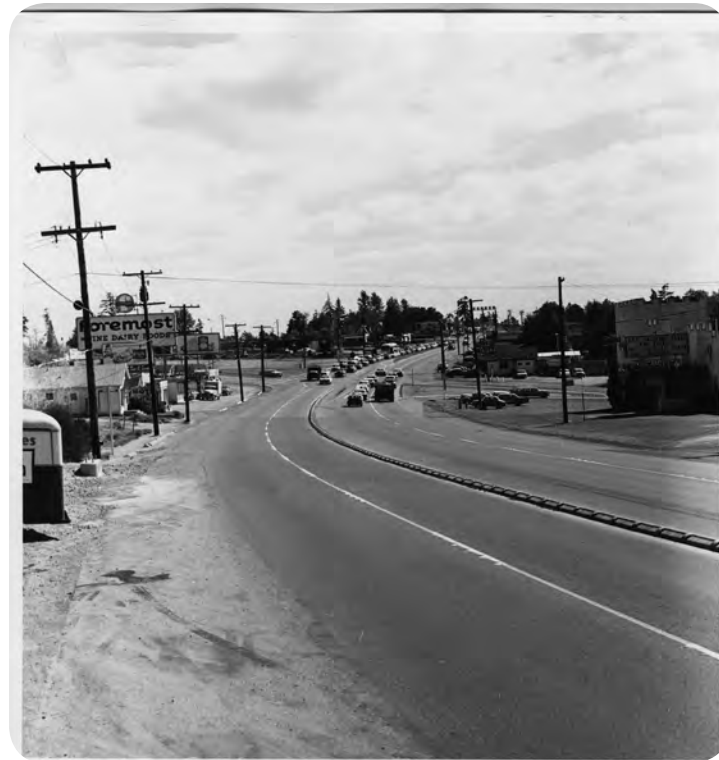
left 1962 view of Primary State Highway 1 (SR 99) at Midway, looking south. Intersection with secondary state highways 5A and 1K. Source: Washington State Archives
