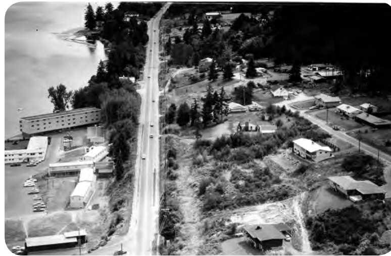
right August 4, 1968, view of Oyster Bay to Chico (SR 3). Source: Washington State Department of Transportation.
