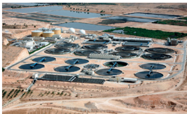
Treating sewage and producing biogas in Jordan 59
