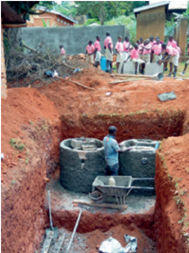
A small community biogas digester being installed in Uganda 9 .
