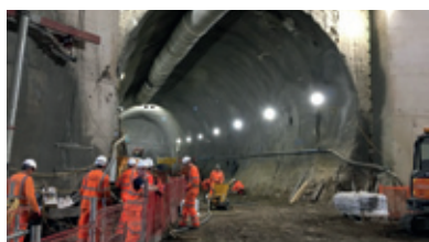
Building the London Super Sewer
