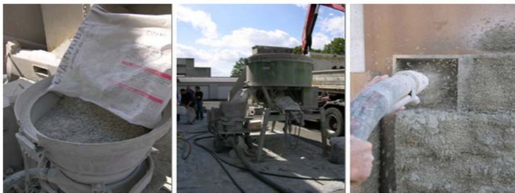
Figure 22: Device for spraying hempcrete (Collet et al., 2013)
