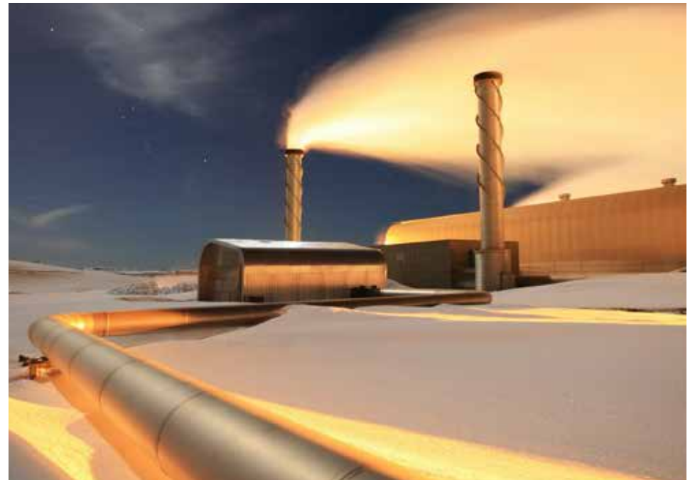
Reykjanes geothermal power plant
