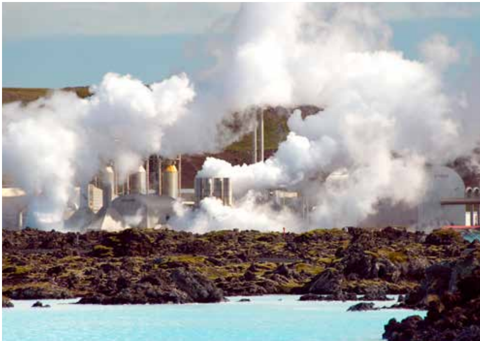
Svartsengi geothermal power plant
