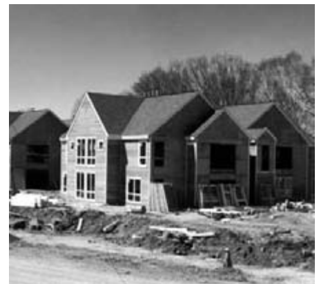
Faculty housing under construction, April 1991
