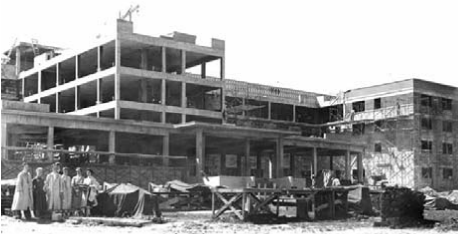
Students pose aside Spellman during construction, 1957
