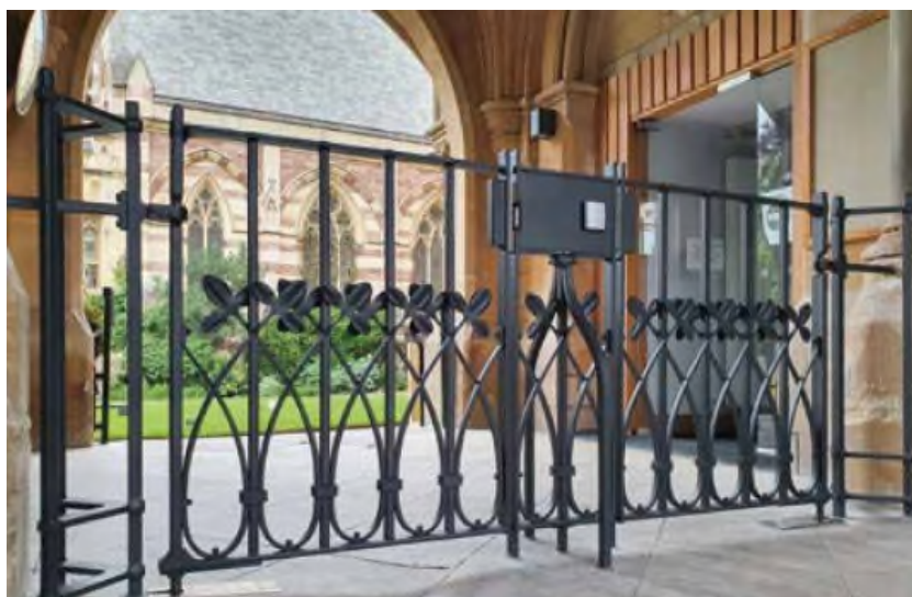
New wrought-iron electronic gates at Broad Street Lodge. Design and photograph by James Price.
