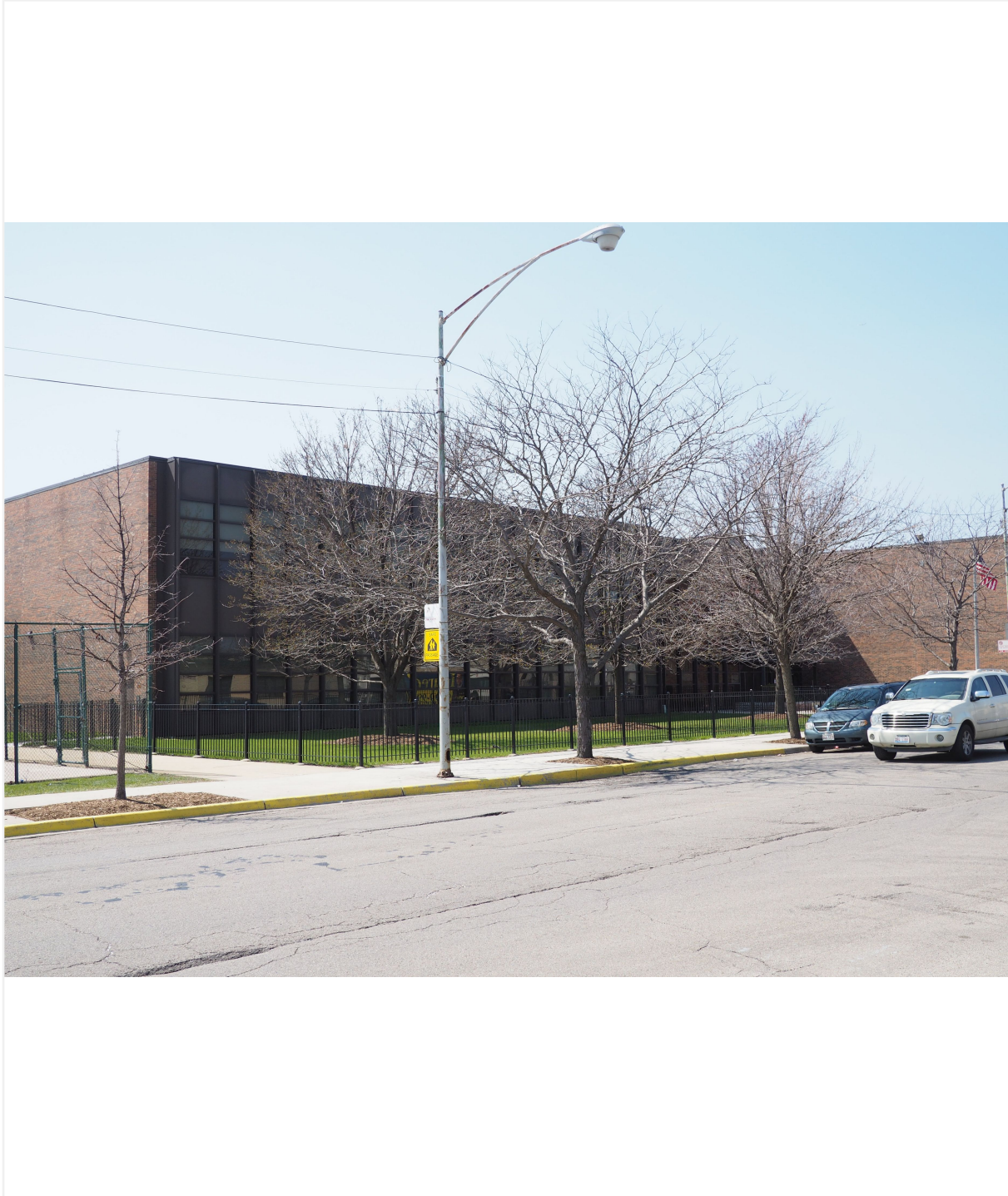
Facing southwest to north-facing facade and east side elevation from West Harrison Street
