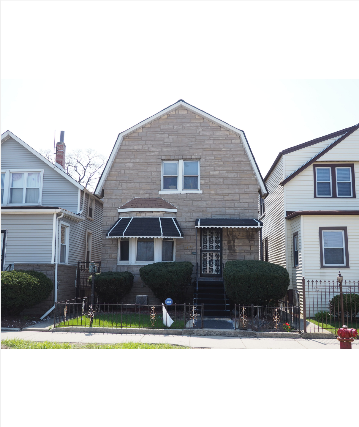
Facing south to 4915 West Lexington Street
