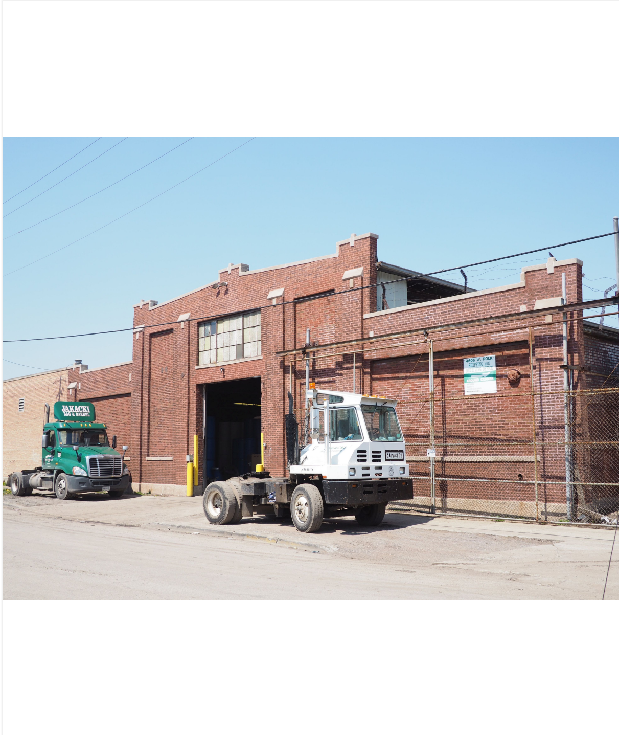
Facing northwest to south rear elevation from West Polk Street
