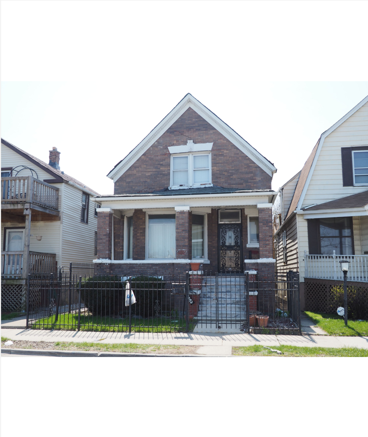
Facing south to 4903 West Lexington Street
