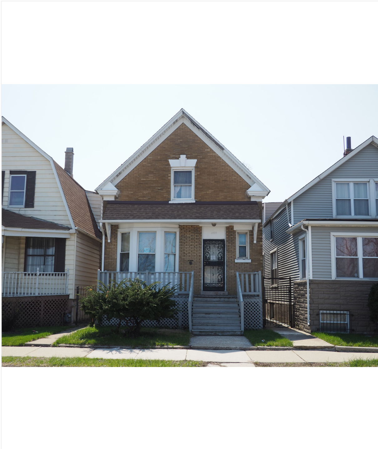
Facing south to 4909 West Lexington Street
