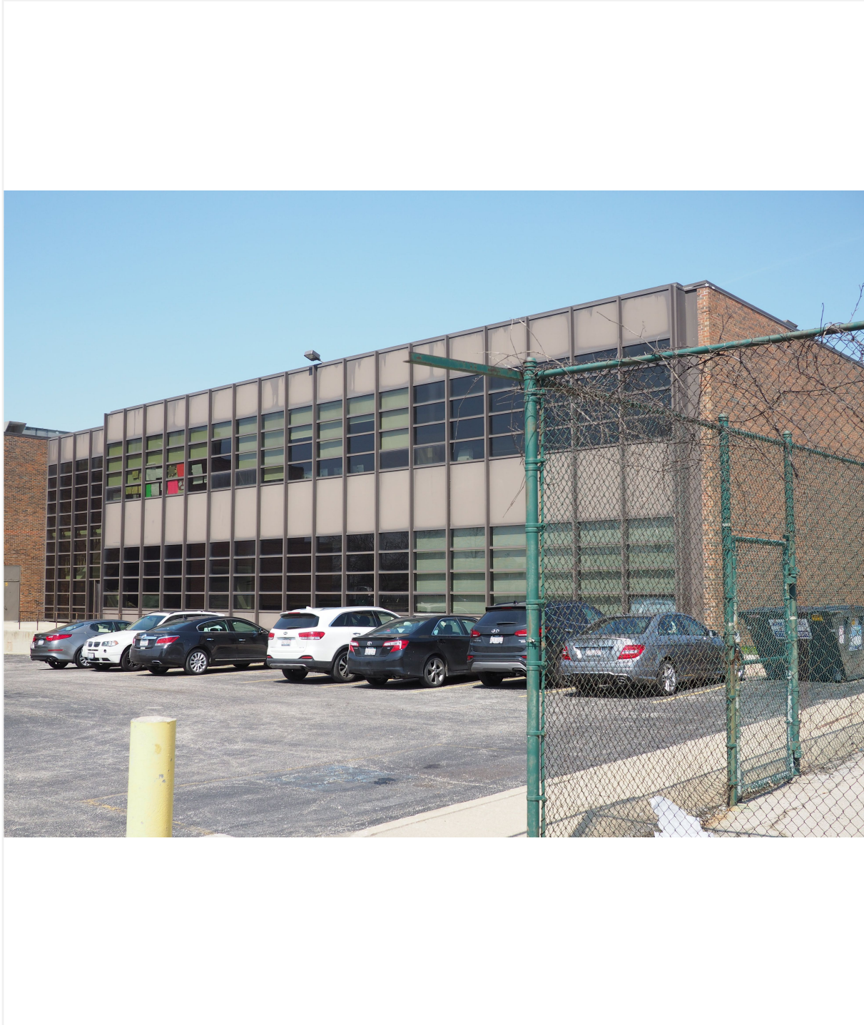
Facing northwest to south rear elevation from West Flournoy Street
