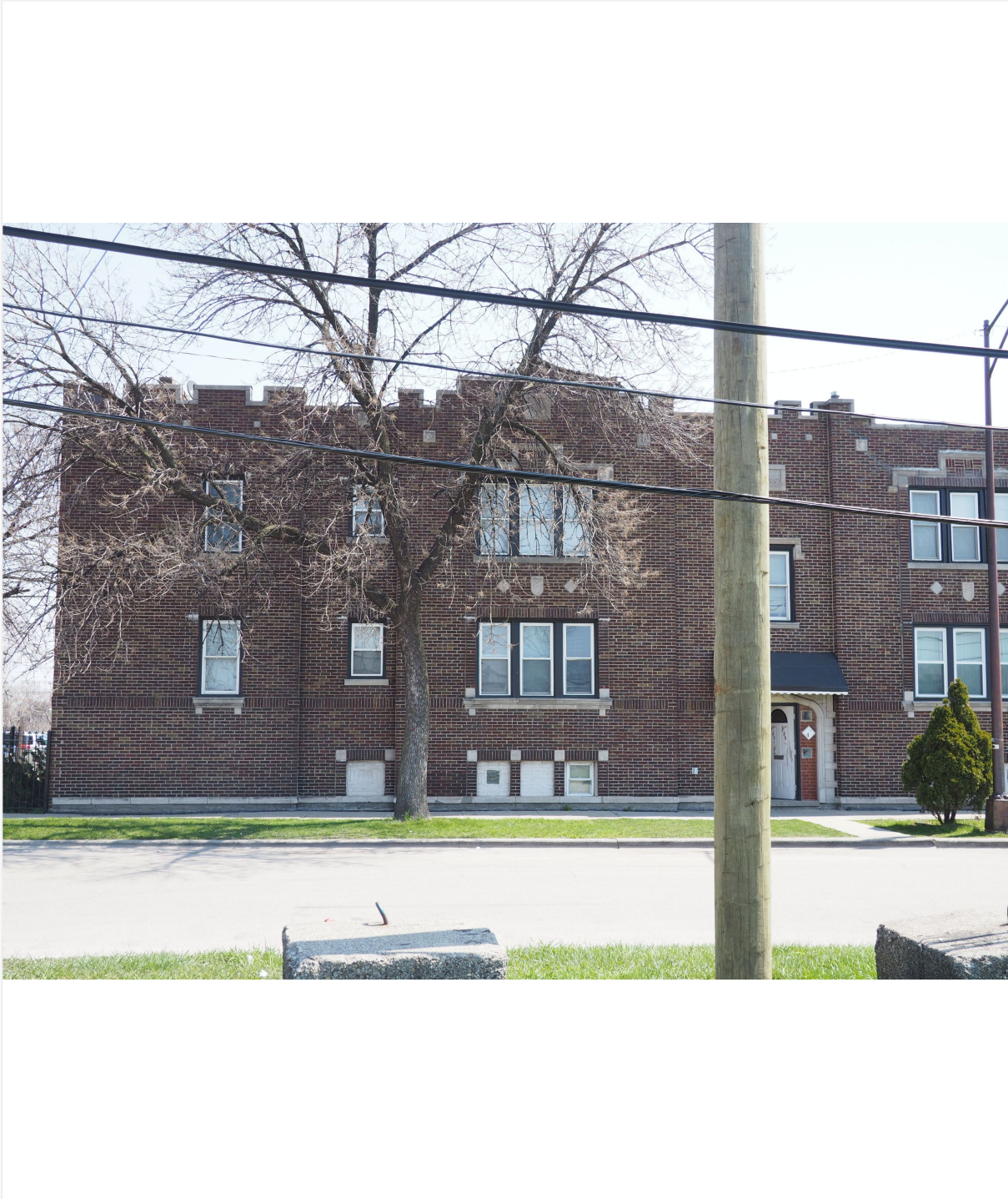
Facing east to west-facing facade of 733 South Lavergne Avenue
