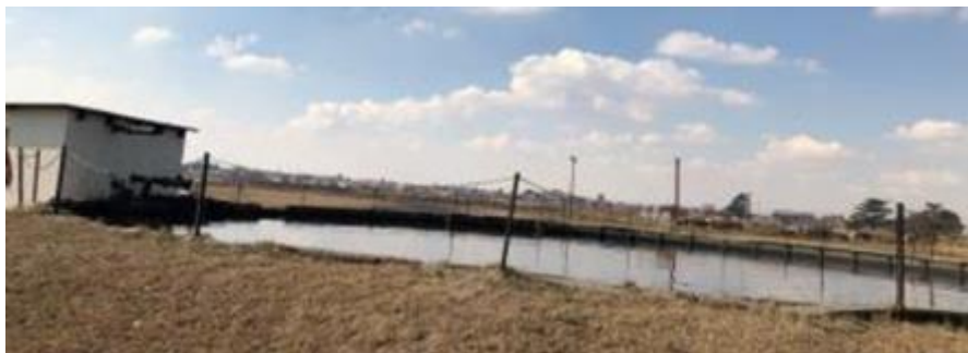
Photograph 2-6: PCD at 3 Shaft
