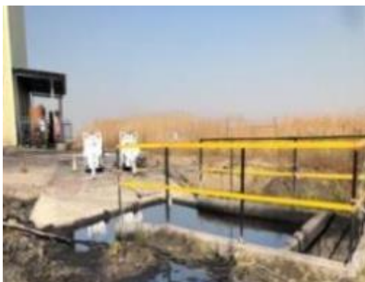
Photograph 2-9: Sump located at workshop
