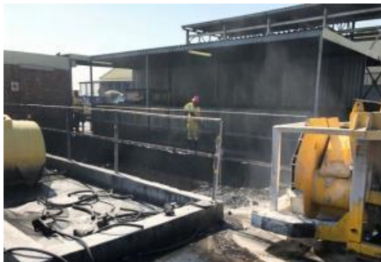
Photograph 2-7: Sump located at wash bay
