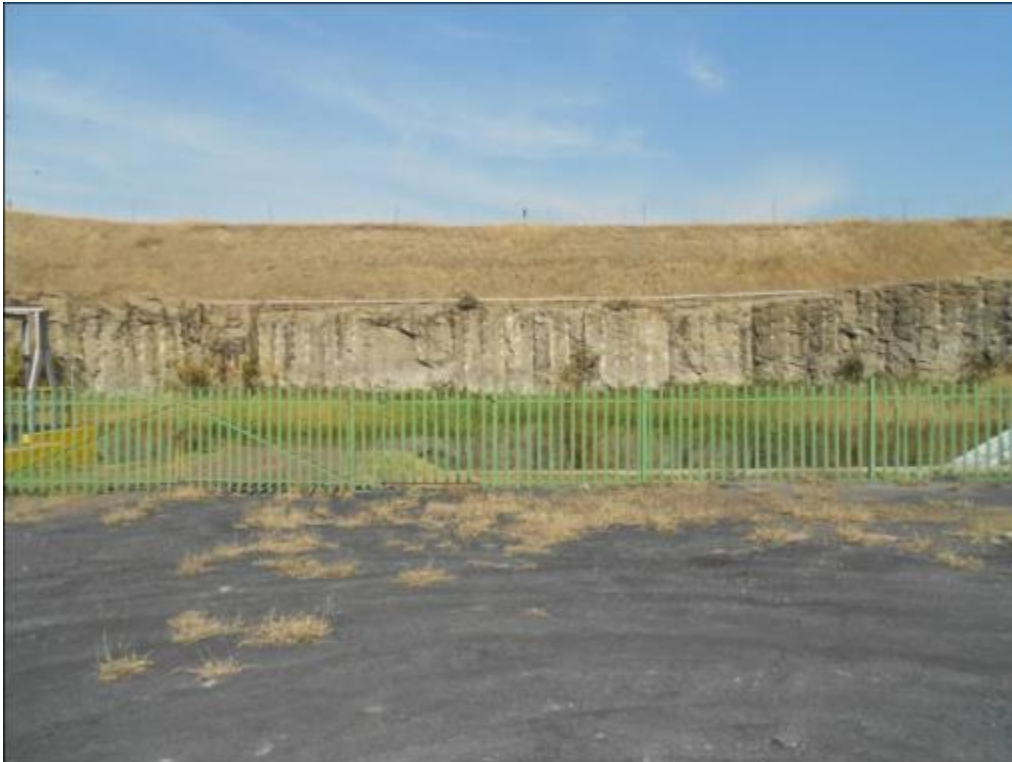
Photograph 7-1: Adit Sump (MK-Pit)
