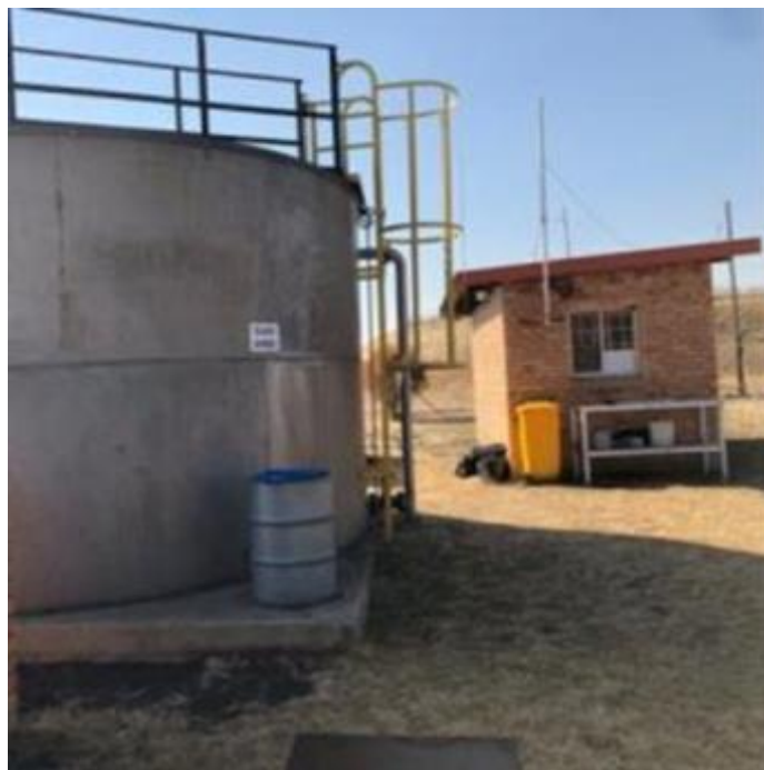
Photograph 2-2: Chlorine tank
