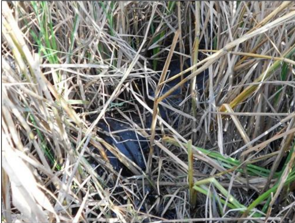
Photograph 7-2: Pipe discharging the sump and underground water (MK-Sump)
