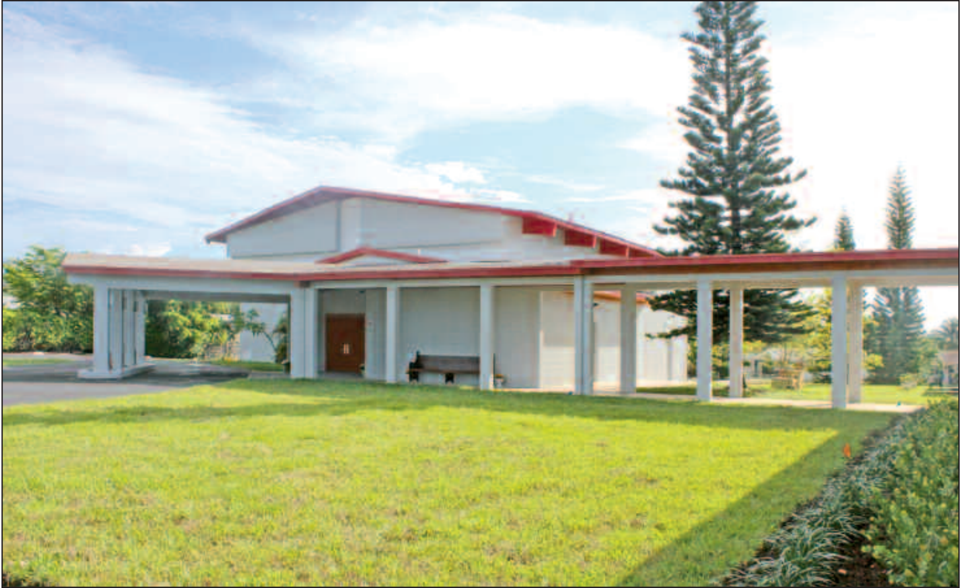
Holy Guardian Angels, Lantana, Florida, U.S.A. celebrated the dedication of its new entrance during Archbishop Haverland's visitation to the parish on Sept. 20. The project includes a new narthex, porte-cochere, columbarium and cloister, and was made possible by a donation in memory of Ann and Kenneth Bachellor, deceased members of the parish. It completes, in a physical sense, the amalgamation of St. Augustine of Canterbury, Holy Spirit and Guardian Angels parish into Holy Guardian Angels Anglican Catholic Church. Art from all three parishes plus the Diocese of Nueva Granada and the former parish of St. John the Theologian, Pompano Beach, Florida adorn the walls of the narthex.
