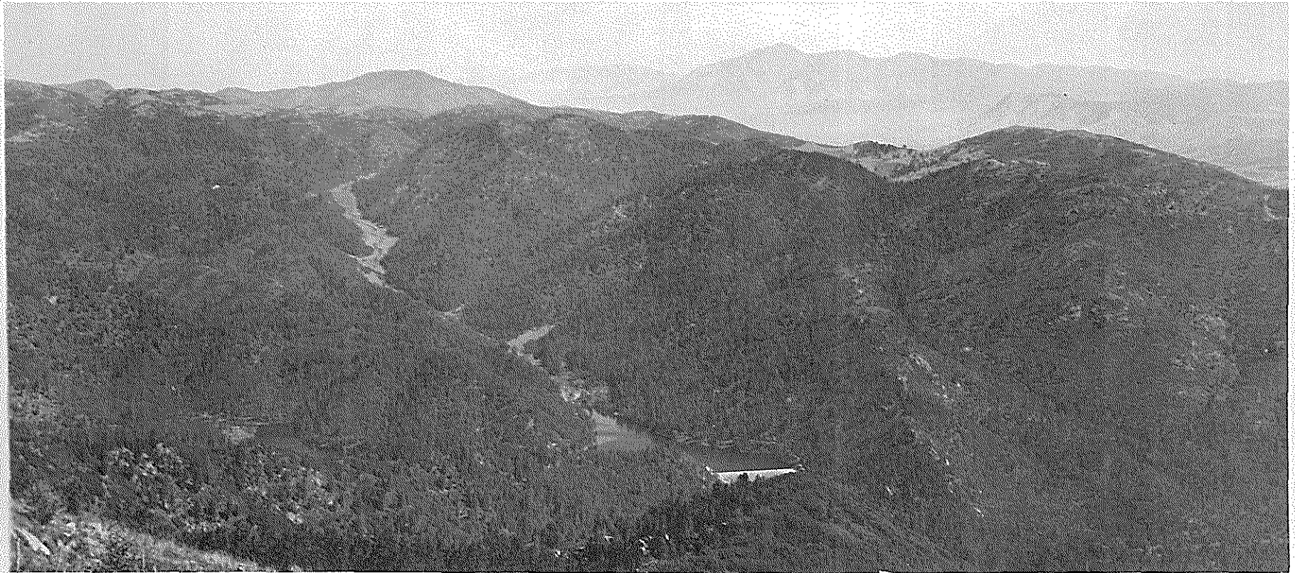
Bonito Dam and Lake on Rio Bonito, a principal tributary of Rio Hondo, high in the massive Sacramento Mountains which form the western rim of the Rio Hondo drainage basin in south-central New Mexico. Developed primarily for railroad uses, the headwater impoundment now serves municipalities in the upper Hondo Valley and in arid Tularosa Valley to the west, bounded by peaks in background (see p. 11-12). View is to the northwest.
