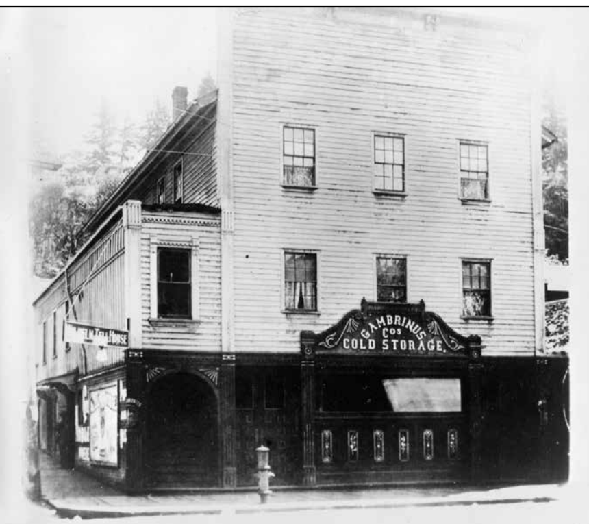
Legislators used this and several other commercial buildings in Salem during the period between the loss of the first and the opening of the second Capitol (1855–1876).
