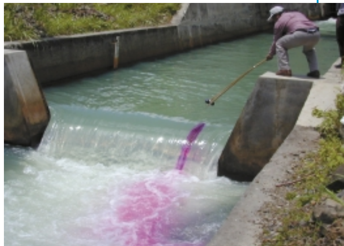
Using an artificial tracer to identify the source of leakage.
