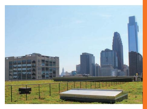
PECO's 45,000 square foot green roof helps reduce storm water runoff and reduce summertime peak roof temperatures up to 80 degrees, saving on heating and cooling costs.
