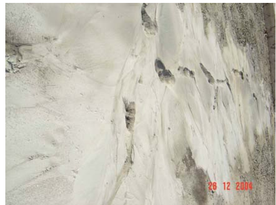
Fig. 3 - Liquefaction at Haddo Wharf, Port Blair, Andaman Island
