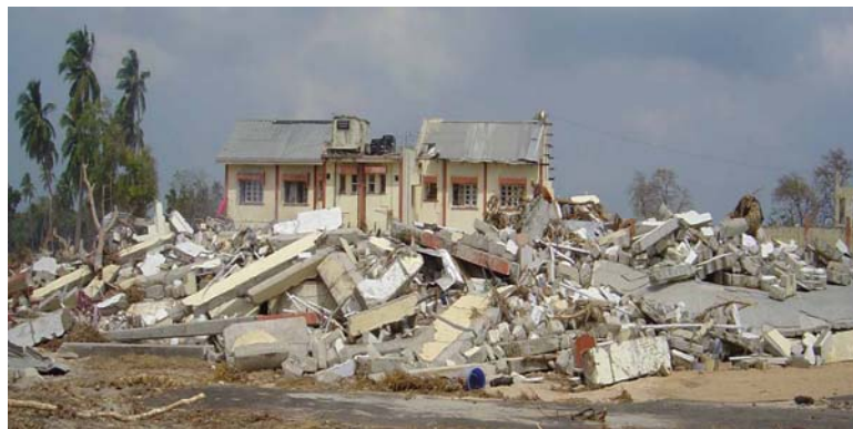
Fig. 4 Collapse of buildings due to tsunami waves
