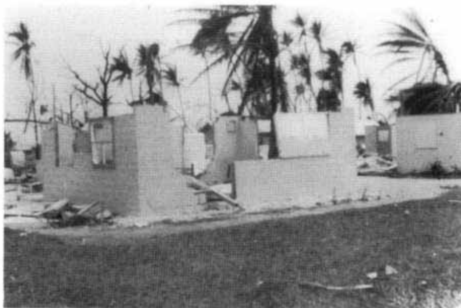
Damage from Cyclone Bebe on Funafuti, Tuvalu, 1972.
