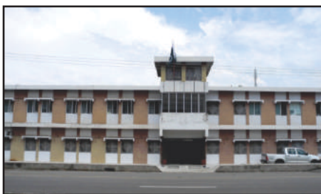
New Building MATRC Islamabad
