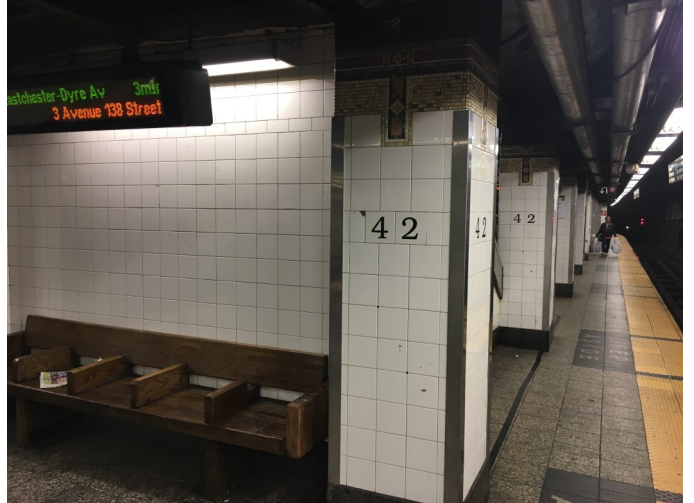
The bulk of P15 is clearly apparent in this photo, looking south, which impedes circulation and creates a visual barrier. May 31, 2018.
