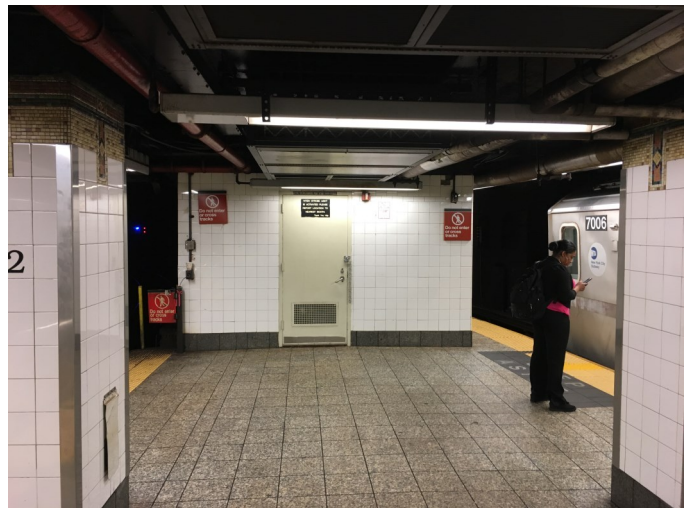
View of the north end of the southbound platform on June 21, 2018. By next year there will be a new stairway here up to the enlarged north mezzanine.
