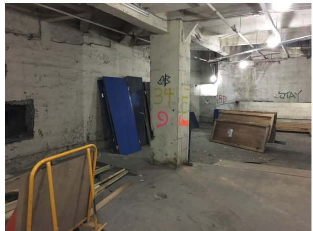
A June 15, 2018 view of the northern basement space reclaimed from the Grand Hyatt Hotel. The wall to the left will be demolished to enlarge the north fare control area.
