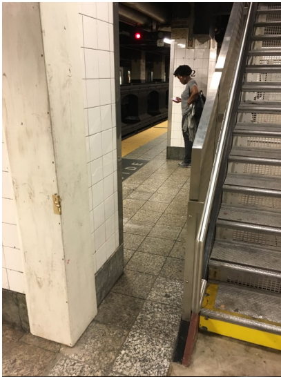
Note the increased clearance on the platform between P24 and the columns, which will facilitate better passenger circulation and enhance safety. June 21, 2018.
