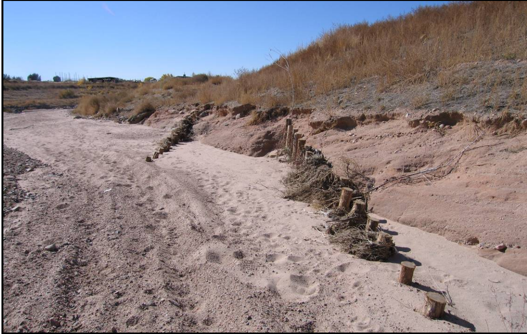
Figure 8.H. Juniper post veins encourage accretion along the channel banks Photo facing downstream Source: photo by author (2008)
