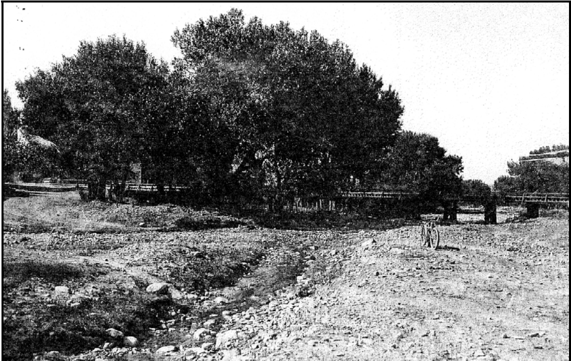
Figure 6.N. Compound channel, 1912 Small, nested stream within wider gravelly floodplain; bridge width indicates the span of large-capacity floods, photo facing downstream Source: Museum of New Mexico, negative #61570
