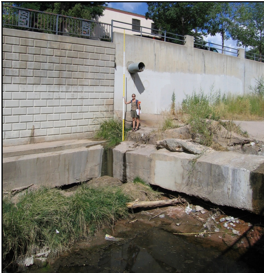
Figure 6.CC. Severe channel incision with reference scale Source: photo by author (2005)
