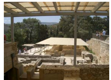
6. Knossos reinforced scarps and steel framed roofs of transparent panels 2005
