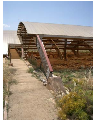
16. Mallia laminated wood arch & polycarbonite roof panels June 2005
