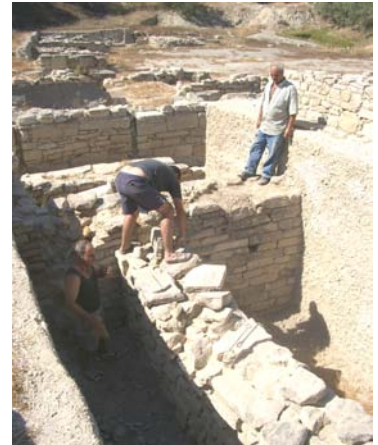
71) Kommos ancient wall stabilization June 2005
