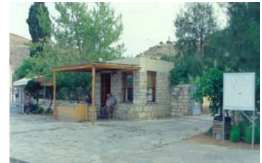
27 Gortyn entrance bldg. July 1997
