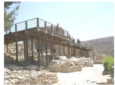
12. Knossos steel & wood walkway 2005
