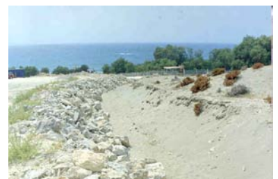
61) Stone line trench, south & east of site August 1997
