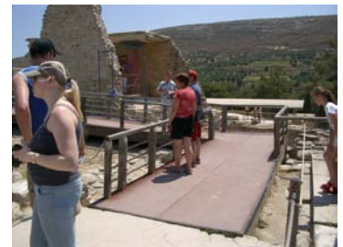
9. Knossos steel & wood ramp walkway 2005
