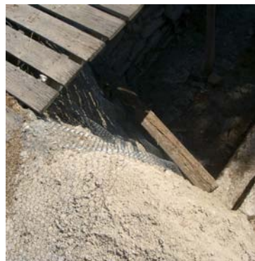
68) Kommos wire reinforcement July 2005
