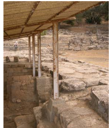
51) Hagia Triada 1985 roof July 2005
