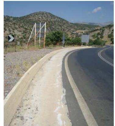
59) Road curb & gutter west of Mallia June 2005
