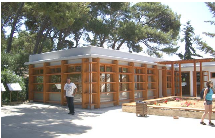
8. Andreas Michelakakis - retail store manager outside the new store outside corner where he would position the entrance door. June 2005
