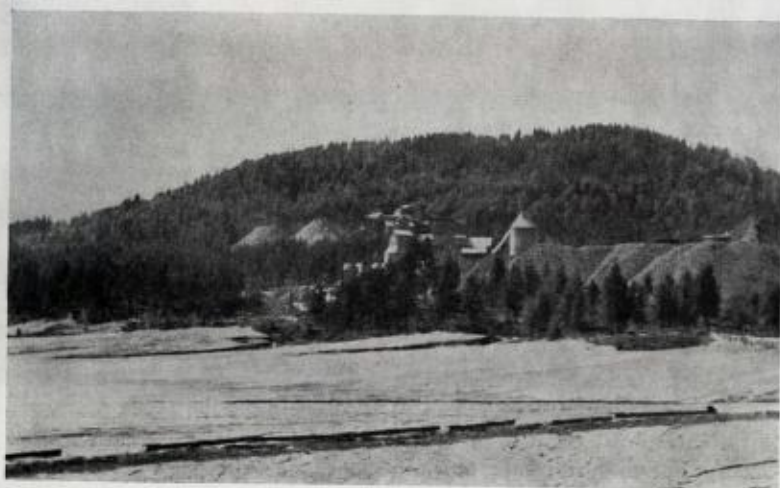
Fig. 1. Flåt nickel mine. From north.
